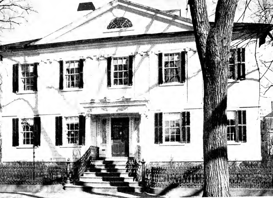
ASSEMBLY HOUSE, SALEM
