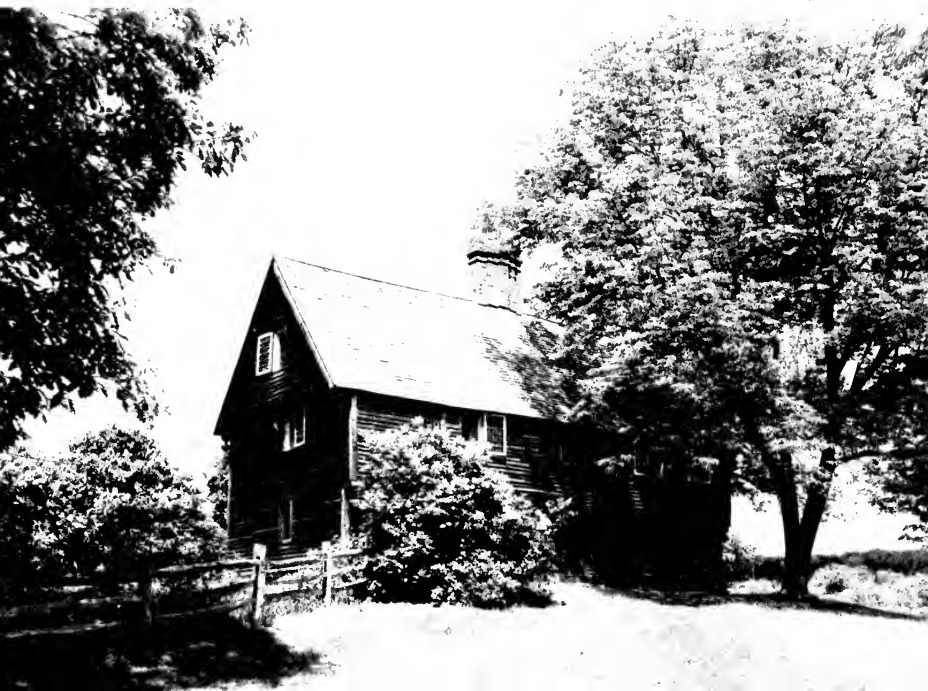
PARSON CAPEN HOUSE, TOPSFIELD
