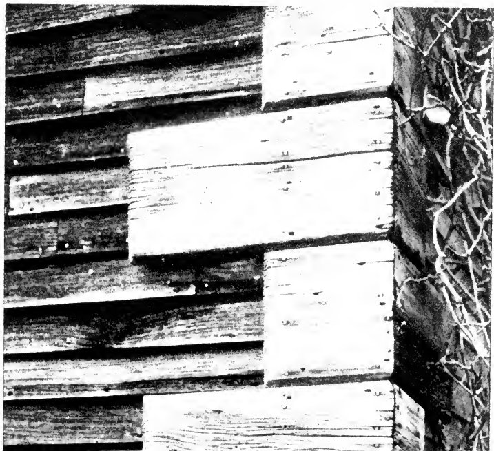
WOODEN QUOINS, WINSLOW HOUSE, MARSHFIELD
