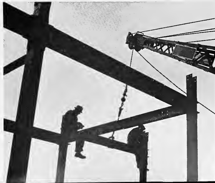
STEEL MEN AT WORK ON NEW DORM—PHOTOGRAPH BY GRANT B. SNYDER
