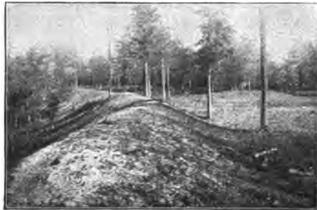
East Wall, North Fort.
