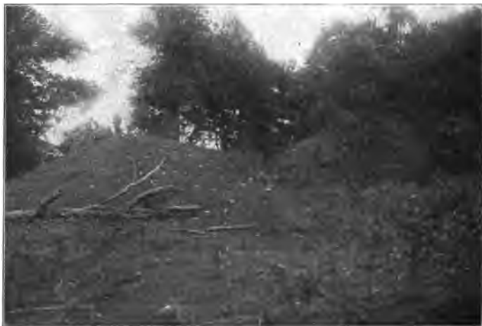
Walls and Gateway — Miami Fort.
