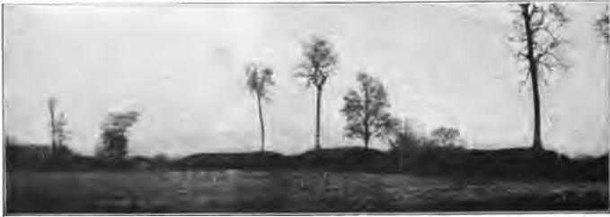
Section of East Wall, North Fort.
