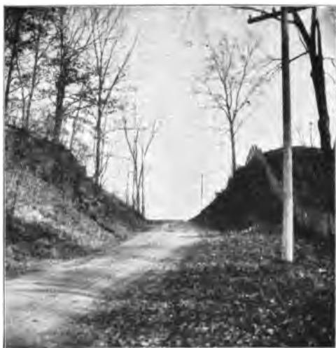
Entrance to Fort from the West.
