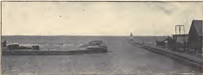
FIG. 60. Piers of Kincardine Harbor, Ontario, looking out.
