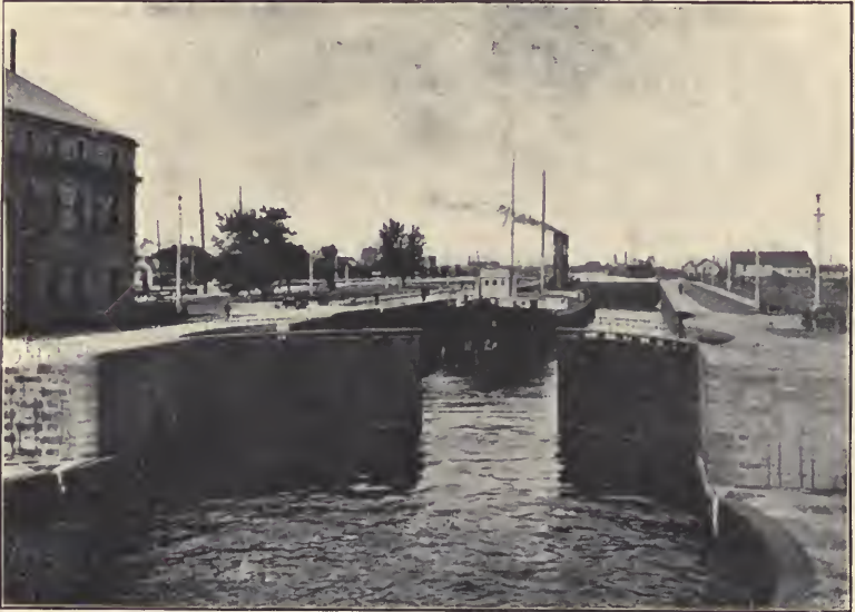
FIG. 58. The American Locks at the Sault Ste Marie. The ship has come from Lake Superior as now she has come down to the level of the river below the rapids, the gates are being opened to let her proceed southward
