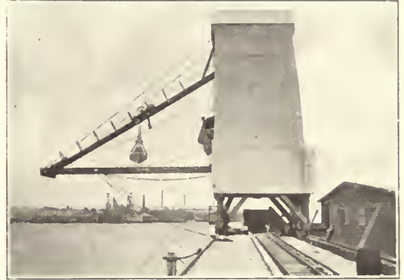
Coal Hoisting Towers.
