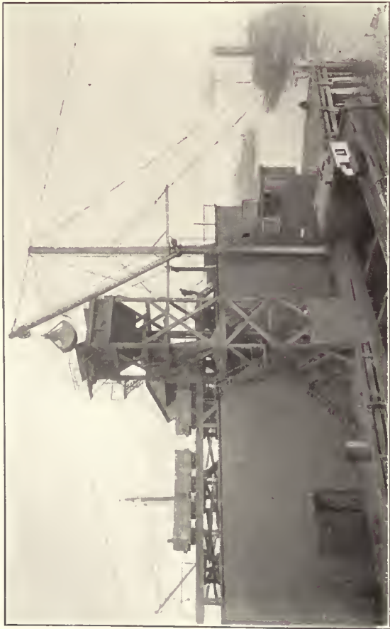
Mast and Gaff Unloader Handling Automatic Grab Bucket
