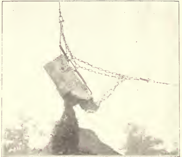
Chain-Bridle Drag-Line Bucket Dumping Loose Material
