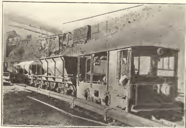
Hopper Bottom Ore Cars
