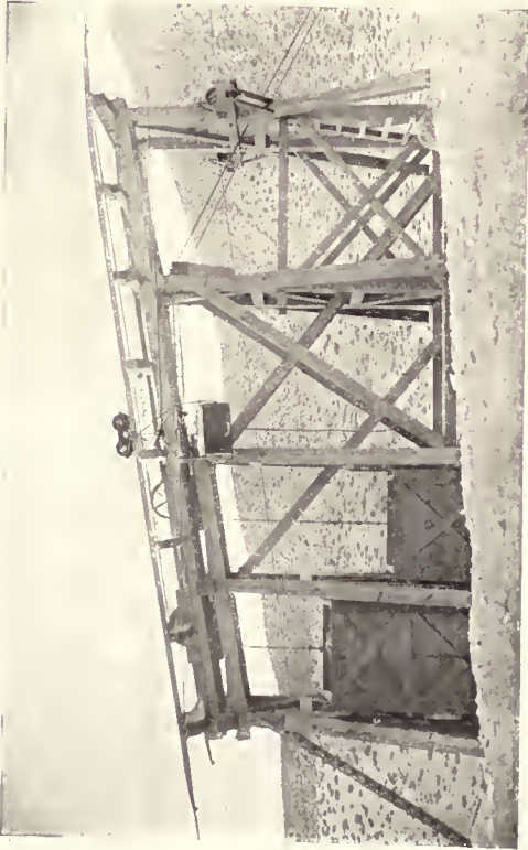
Cable Tramway—Tension Station
