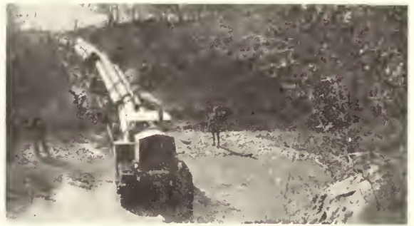
Holt "Caterpillar" hauling 36 tons of casing direct to location
