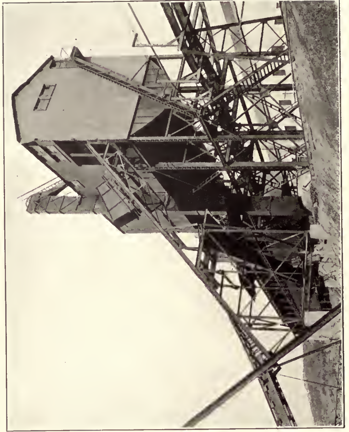
Skip Cars Hauling Coal to Overhead Bunkers
