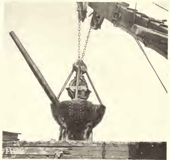
Vulcan Orange-Peel Dredging.
