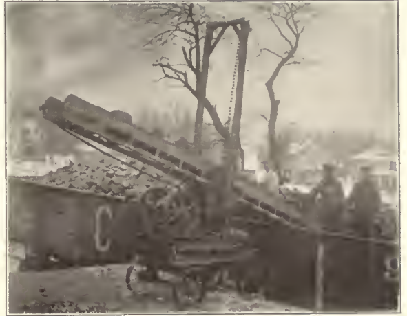
Portable Coal Unloader and Loader Handling Coal from Gondola to Trucks.
