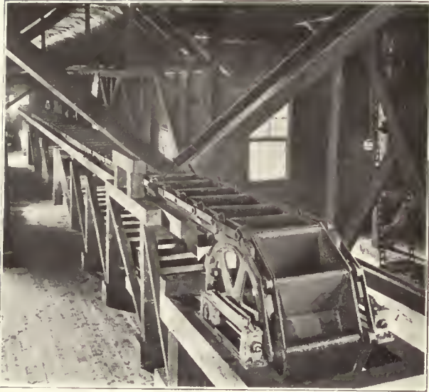
Corner Turn and Feeding Chutes
