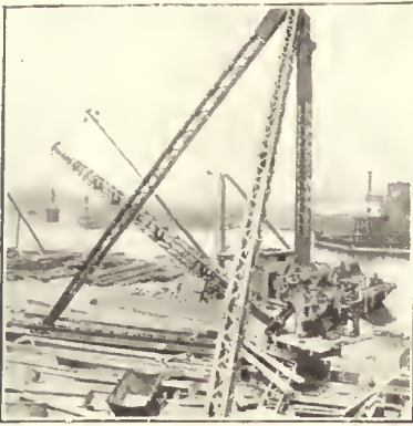
5-Ton Self Slewing Derrick.
