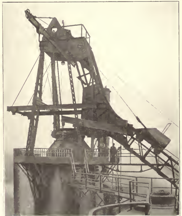
Blast Furnace Skip Car
