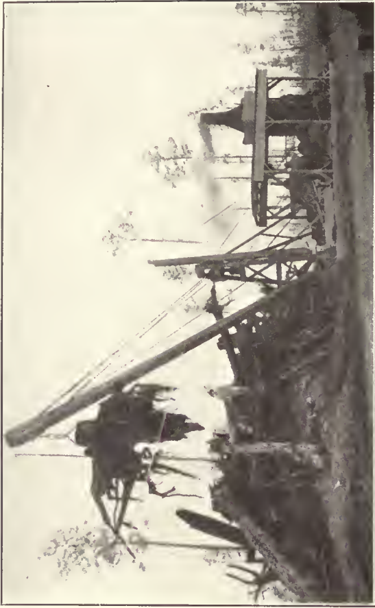
Steam-Operated Stump Puller for Clearing Cut-Over Land
