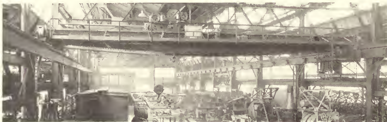
P & H 15-ton crane with 3-ton auxiliary. Chain Belt Co., Milwaukee.
