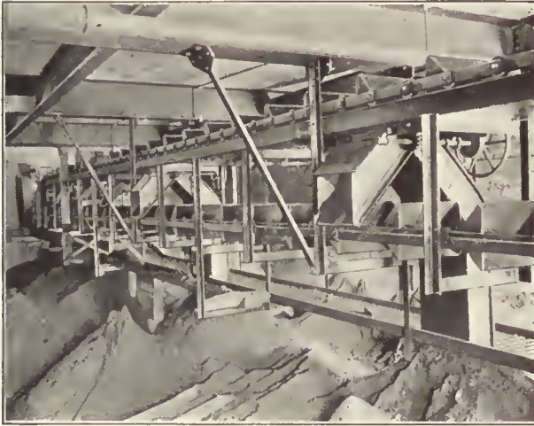
Discharge Chutes on Upper Run
