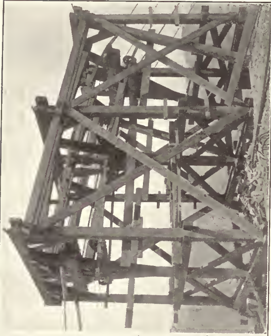
Cable Tramway—Breakover or Rail Station
