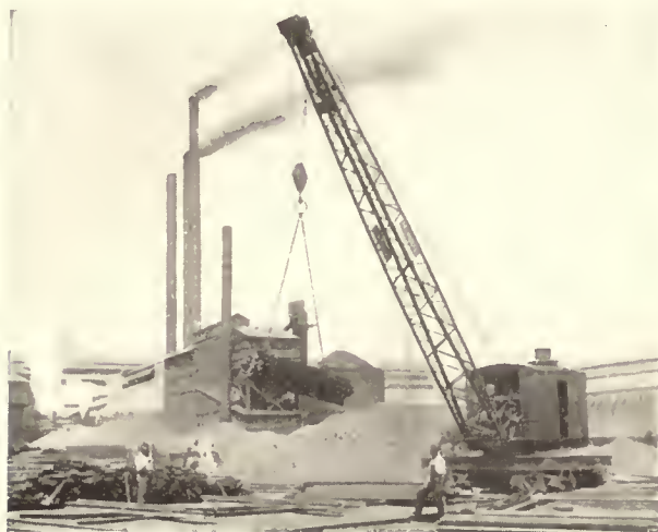
Brownhoist No. 4 Steam Locomotive Crane, Mounted on Standard M. C. B. Trucks, Handling a Bundle of Rails at a Steel Mill.
