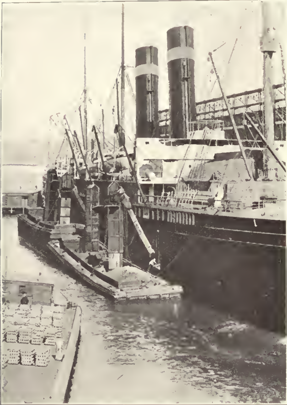
The Discharge Is Through Telescopic Chutes
