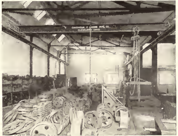
Piling Castings with C-M Crane, Cyclone Hoist and Matchless Trolley.
