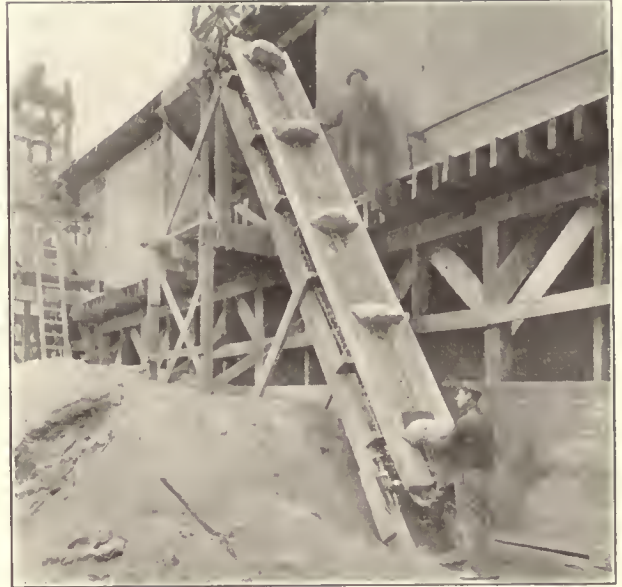
Delivering Cement by Temporary Elevator
