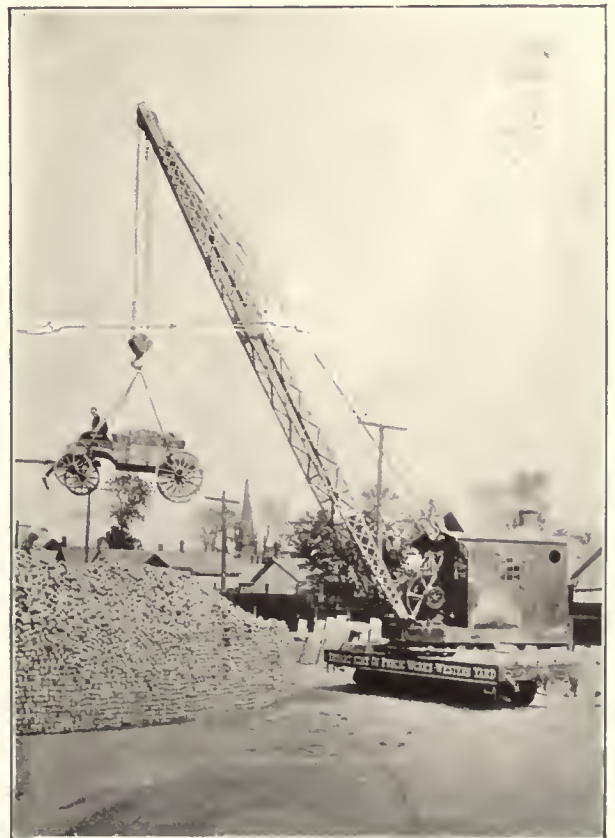
Steam Locomotive Crane Handling Paving Blocks in Dump Wagon with Fall Block, Hoisting Hook, and Chain Grab Hooks
