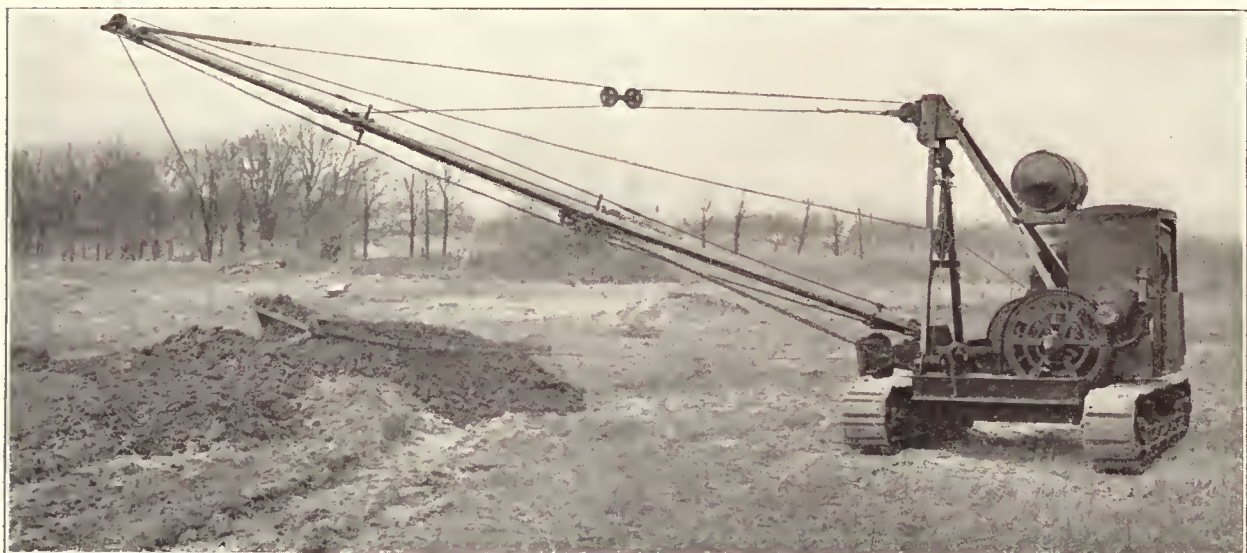
Boom Type Back-Filler Equipped with Complete Creeper Traction
