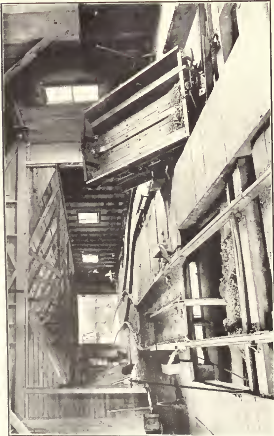
Fig. 1. Cross-Over Car Dump
