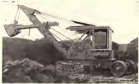
P & H Type 205 Excavator-Crane with Shovel Attachment.
