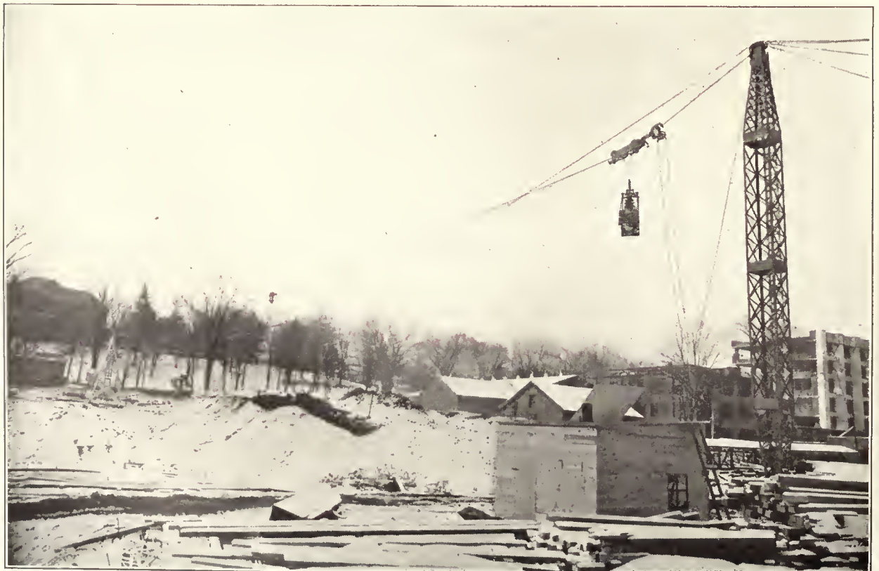
Single Rope Cableway Equipped with Single Line Automatic Grab Bucket for Handling Loose Material
