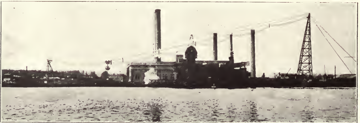
Endless-Rope Suspension Cableway Handling Coal at a Power House with an Automatic Grab Bucket
