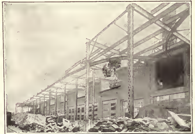
Electric Hoist Cage Control
