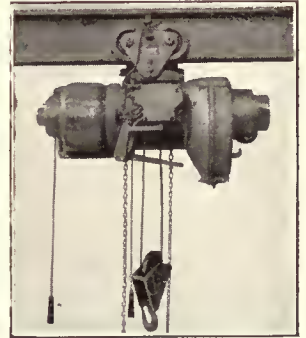
Electric Hoist with Plain Trolley.
