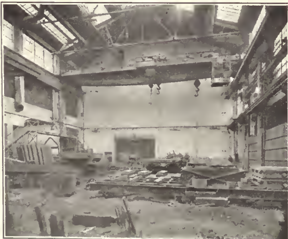
60 Ton Shaw Crane in Foundry.
