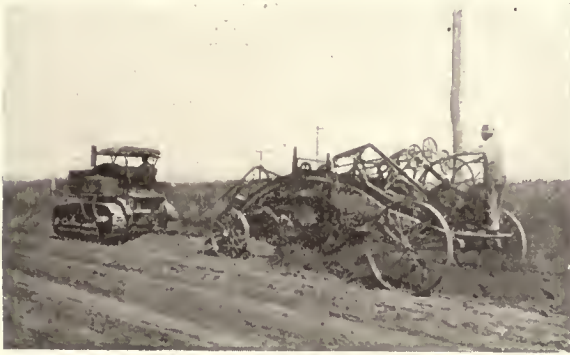
Holt "Caterpillar" Power Is Ideal for Pulling Road Machinery.
