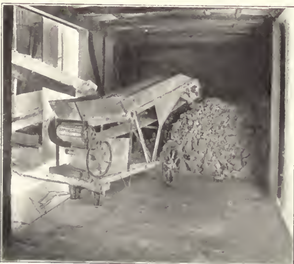
Belt Conveyor Box Car Loader
