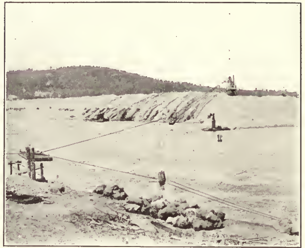
Dragline Scraper Cableway Excavating from River Bed
