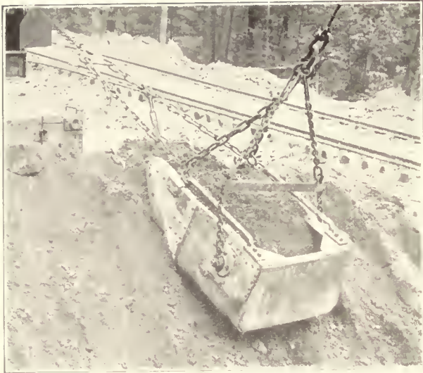
Chain-Bridle Drag-Line Bucket Digging Loose Material
