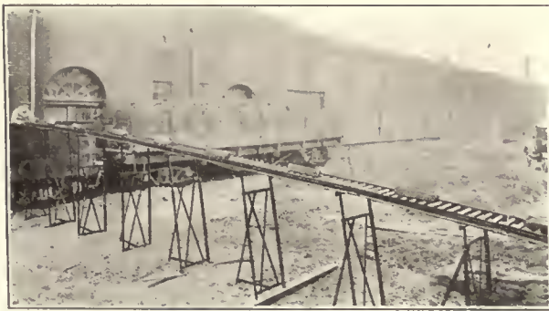
Steel Rollers Are Used for Handling Rough Material
