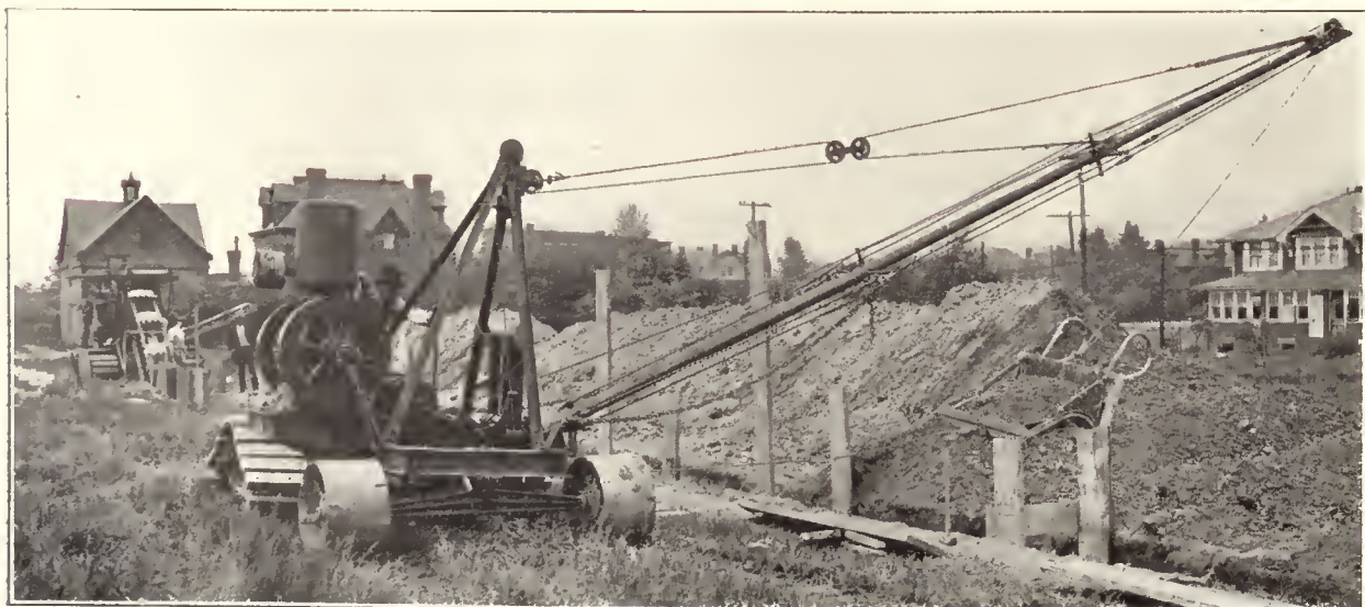
Boom Type Back-Filler Equipped with Plain and Creeper Traction
