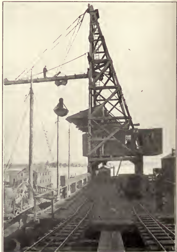
Coal Handling Tower at Power Plant
