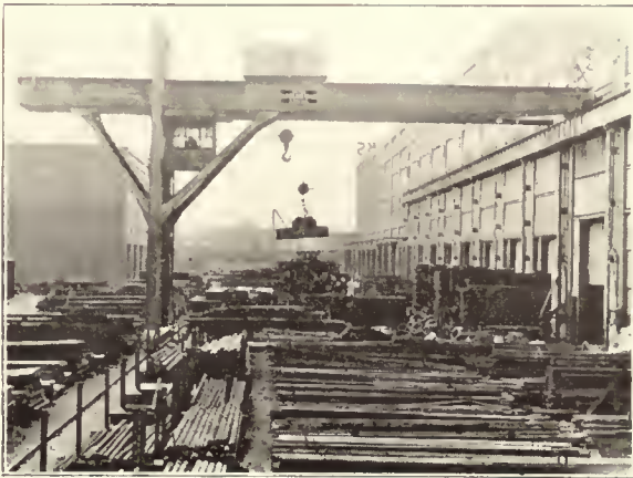
20-Ton Crane in Yard. 1 Leg Gantry.
