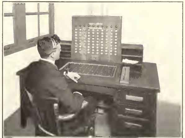
Central Dispatch Board for a group of ten elevators— United States Army Base, Brooklyn.
