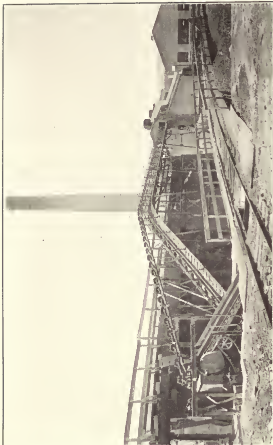
Fig. 7—A Typical Layout Equipped with Flight Conveyors
