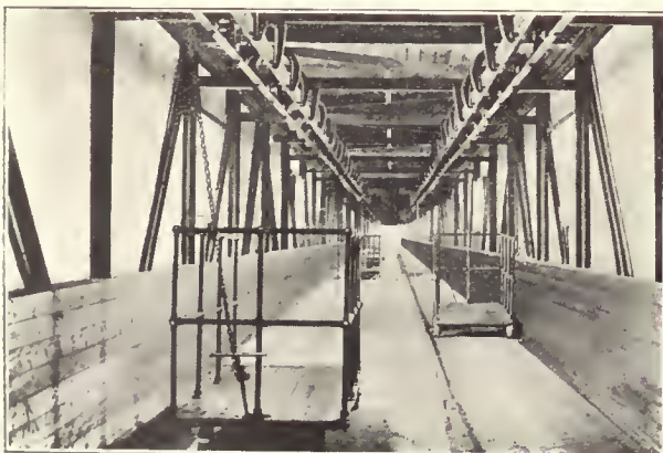
Hauling Trucks by Overhead Conveyor
