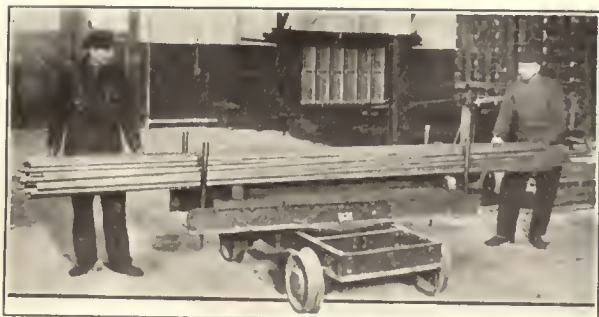
Swivel Top Car for Rods
