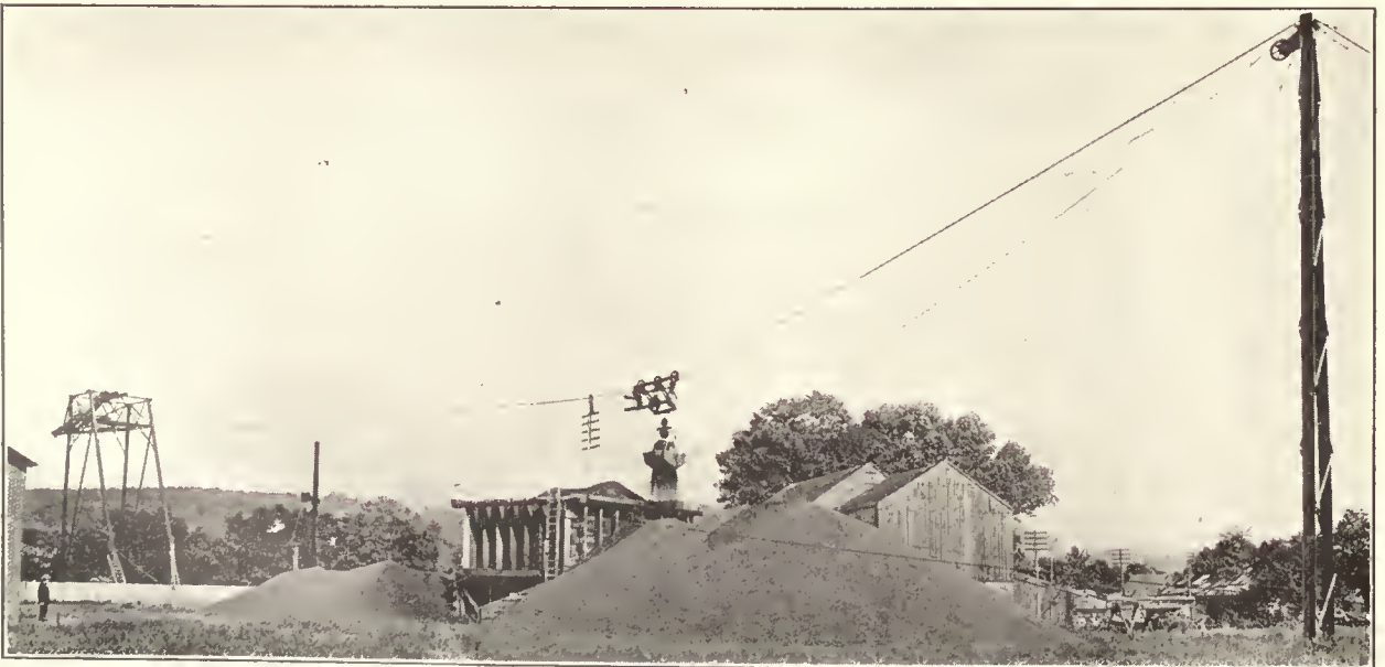
Suspension Cableway with Projecting Boom on Head Tower for Unloading Loose Materials from Boats
