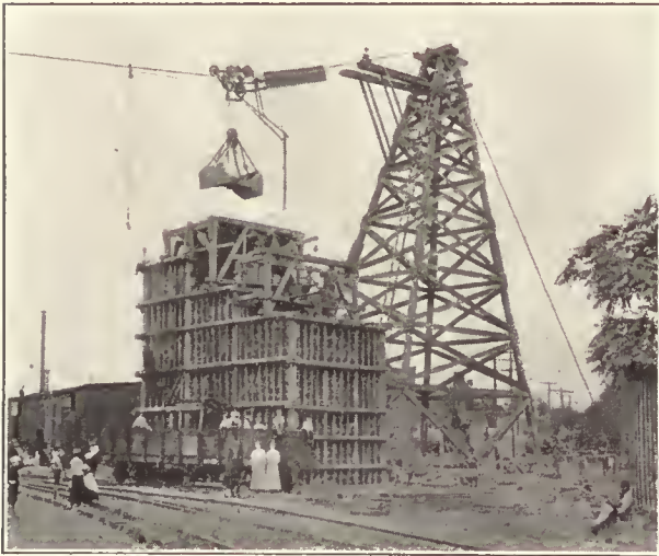
Head Tower and Sand Bin
