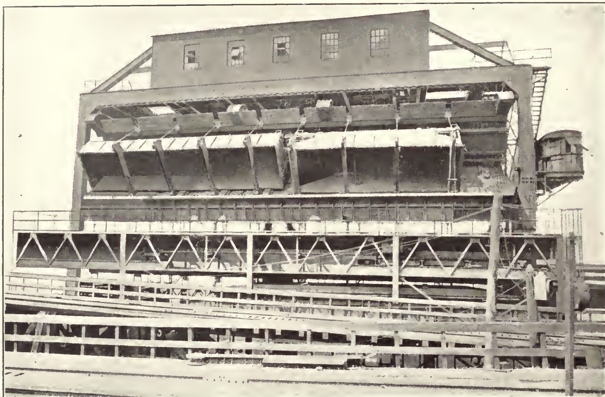
Tandem Car-Dumper with Two Cars in Dumping Position
