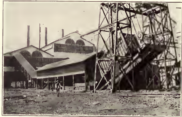
Cane Car and End Dumper
