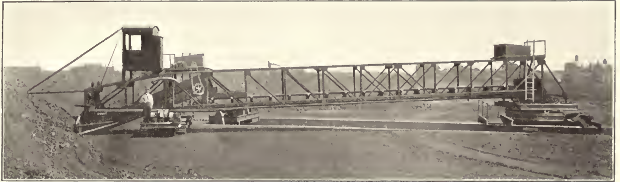
Fig. 17—A Pivoted Bridge Carries the Reclaiming Conveyor
