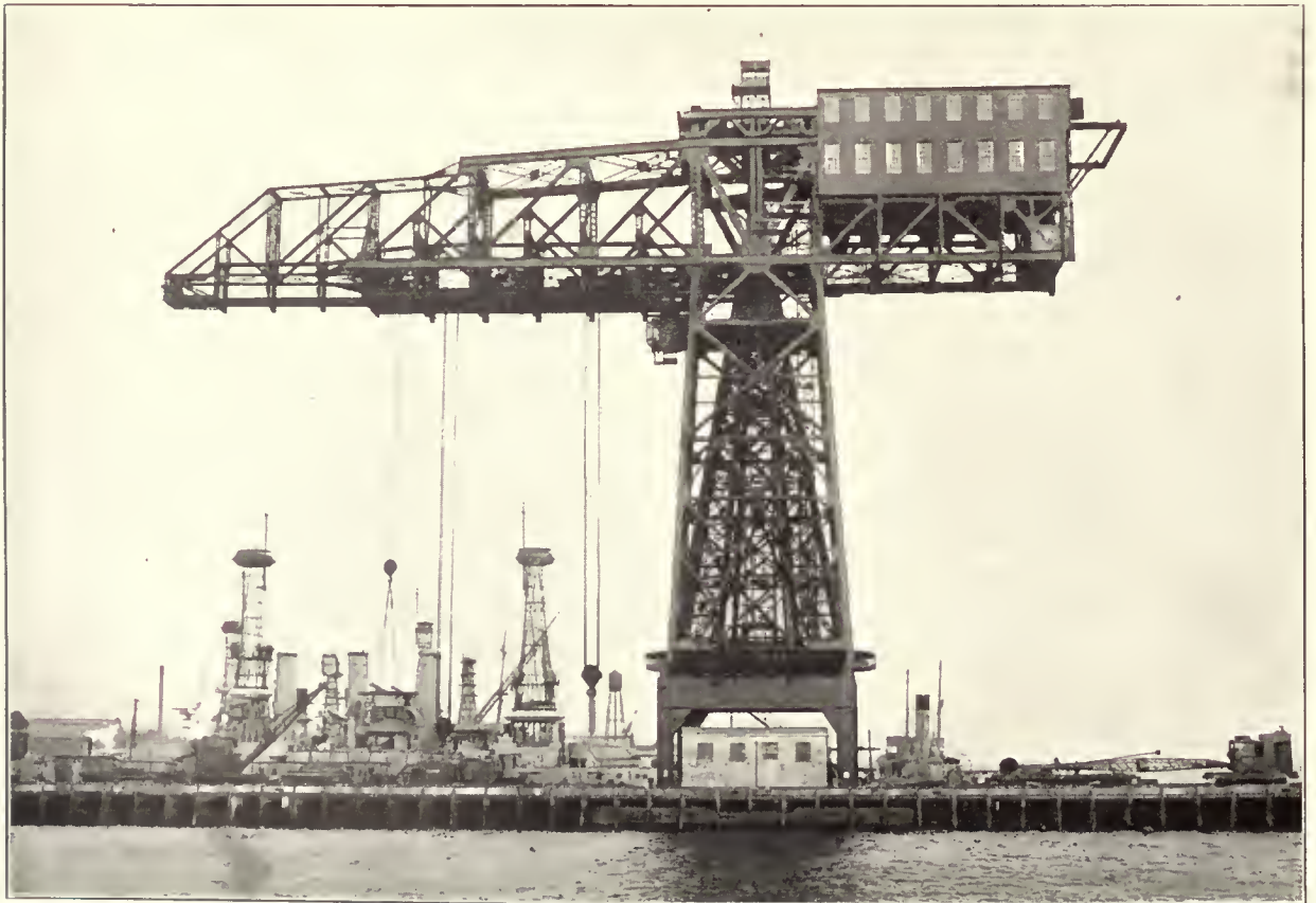
Stationary Hammerhead Portal Crane Installed in Philadelphia Navy Yard. Capacity 350 Tons at 115 ft. Radius; 50 Tons at 90 ft. Radius. Overall Height, 230 ft.
