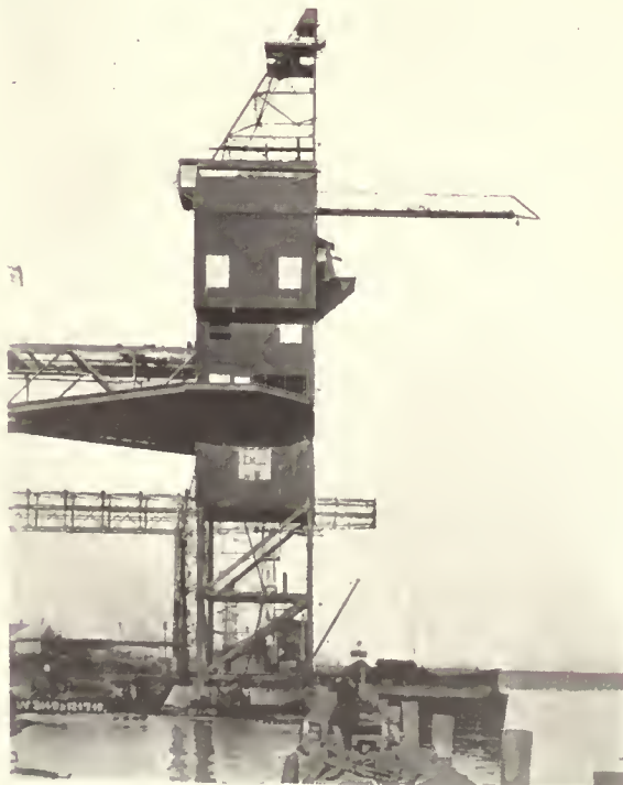
Electrically Operated Tower Unloading Bulk Material.
