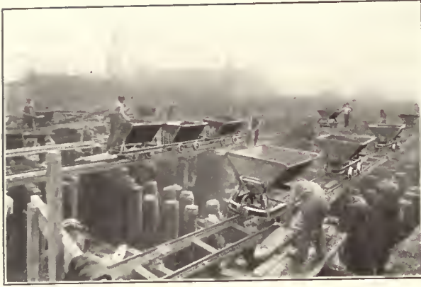
V-Body Dump Car in Construction Work
