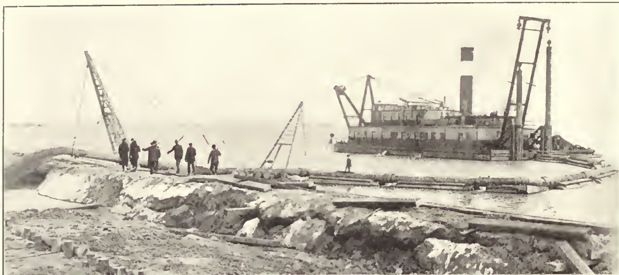
Hydraulic Dredge with Vertical Spuds. Disposal Pipe Line Laid for Filling Behind Bulkhead
