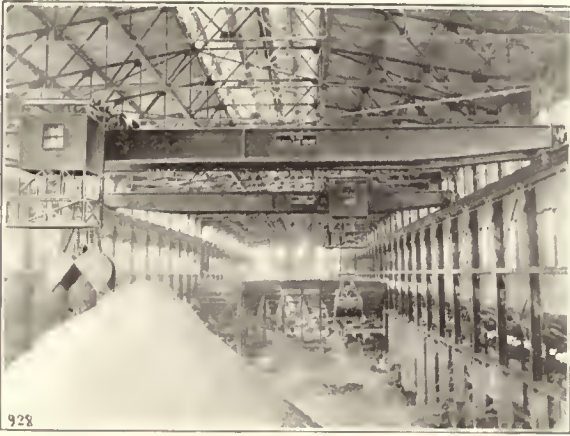
10-Ton Crane Lifting Fertilizer.
