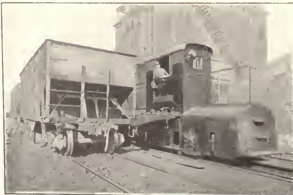
Electric Locomotive, Pusher Type
