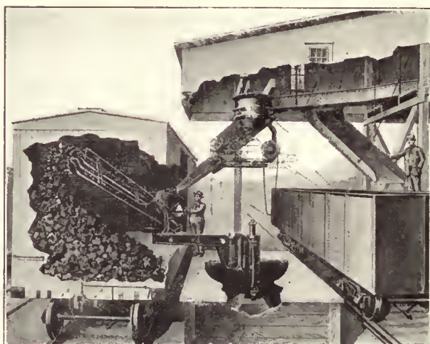
Belt Loader Fed by Double Acting Chute
