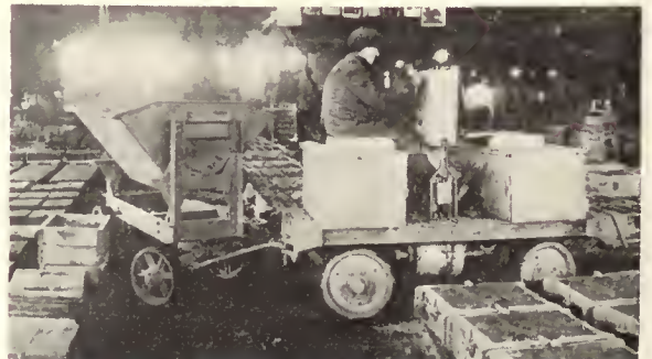
G-E Equipped Electric Tractor Handling Foundry Sand
