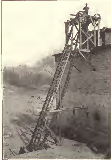
Centrifugal; Perfect Discharge; and Continuous Bucket Elevator
