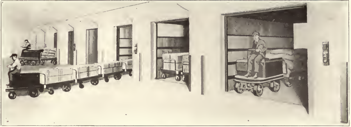
Group of ten Otis Operatorless Elevators in the United States Army Base, showing tractors and trailers unloading from an upper floor.
