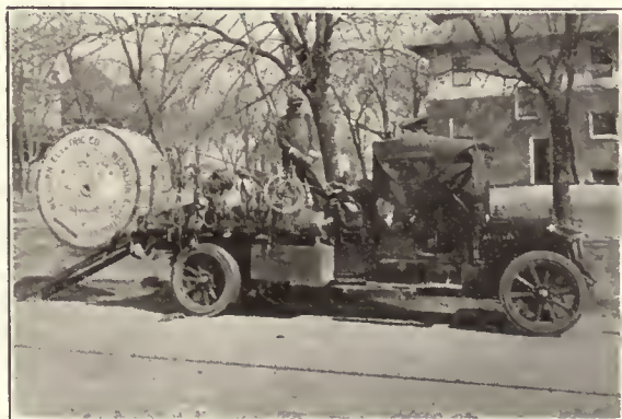
Handling of wire and cable is a simple task with White winch equipment on the 2-Ton truck.
