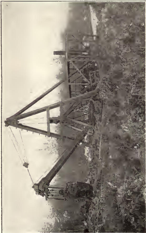
Boom Dredge—Barge Derrick—Equipped with Bull-Wheel and Automatic Grab Bucket
