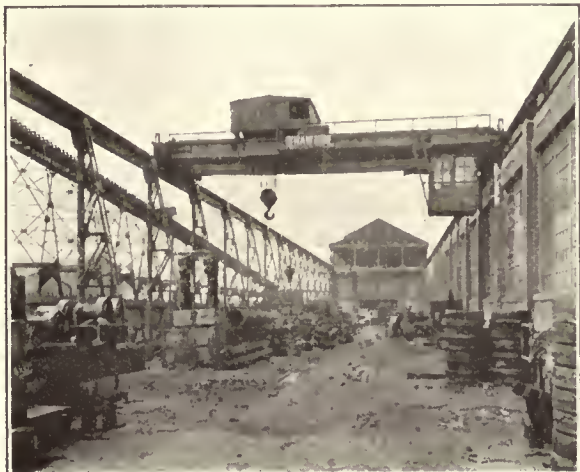
30 Ton Shaw Yard Crane Outside of Shop.
