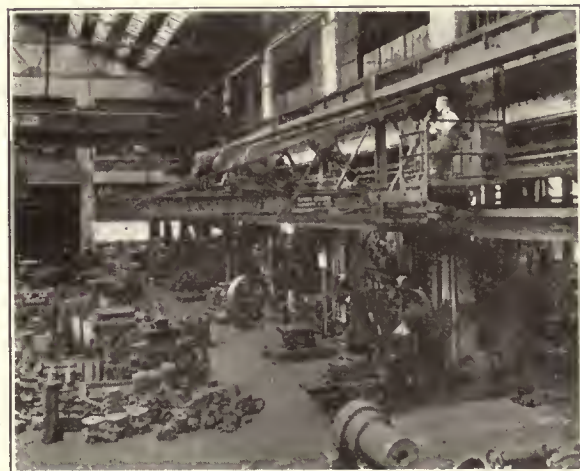
Shaw Wall Crane in Machine Shop.
