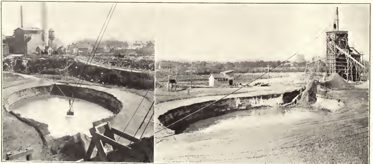
Dragline Scraper Cableway Digging Sand and Gravel from Under Water and Dumping Into Disposal Bin
