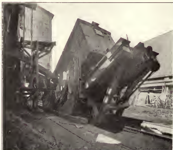
Tilting Box Car Loader
