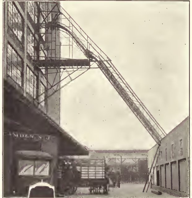
Connecting Operations in Different Buildings
