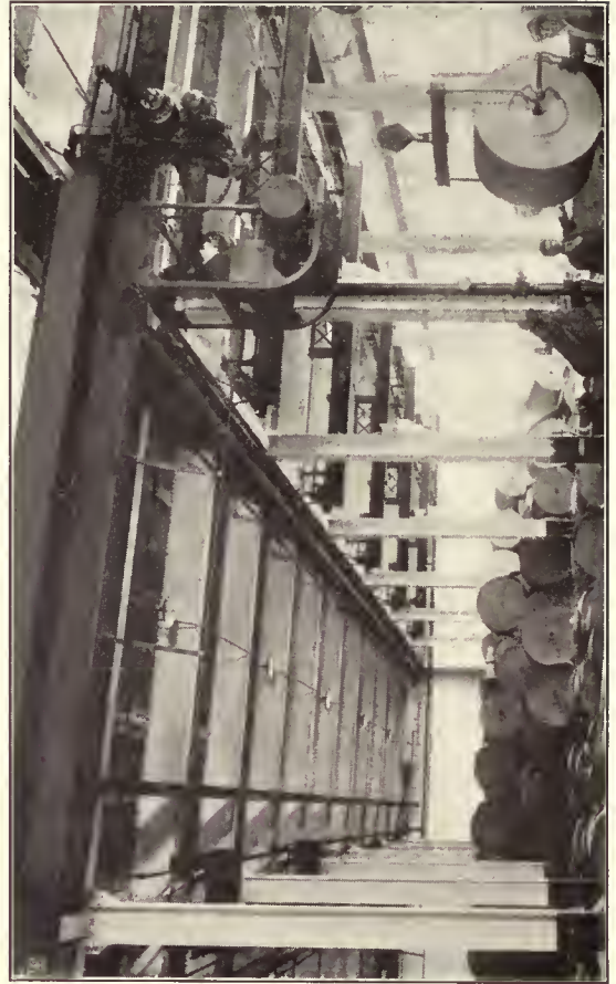
Electric Monorail Hoist Handling Rolls of Paper
