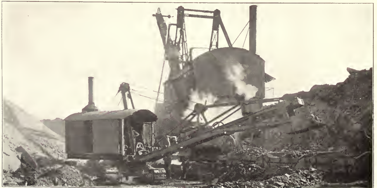
Skimmer or Coal Loader Working in Conjunction with Large Revolving Steam Power Shovel
