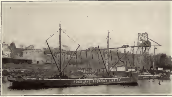
Automatic Railway Handling Stone
