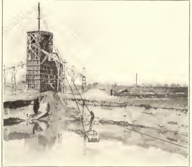
Excavating Gravel from Under Water and Conveying to Screening Plant.
