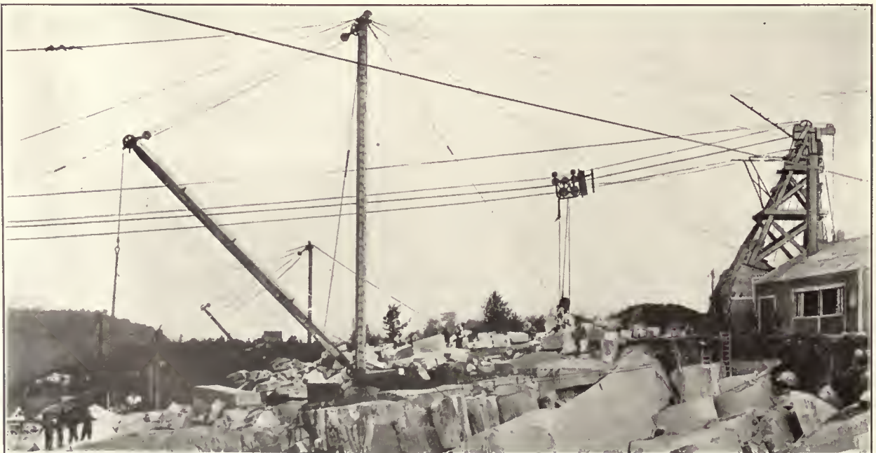
Endless-Rope Suspension Cableway Handling Block Stone in a Quarry
