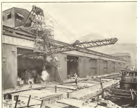
Shaw Wharf Crane Loading Barges.
