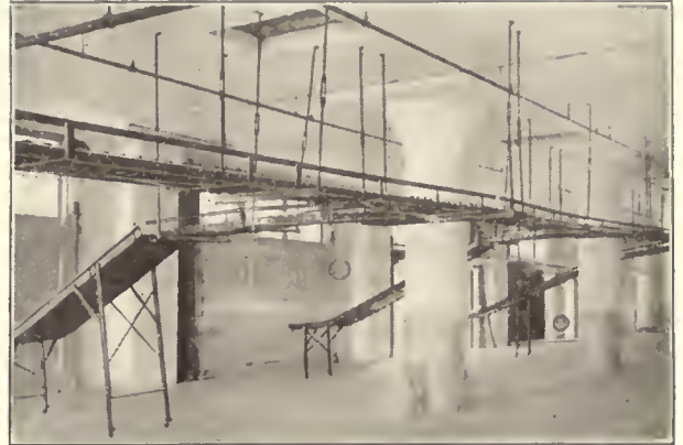
Switches Divert Packages to Cars
