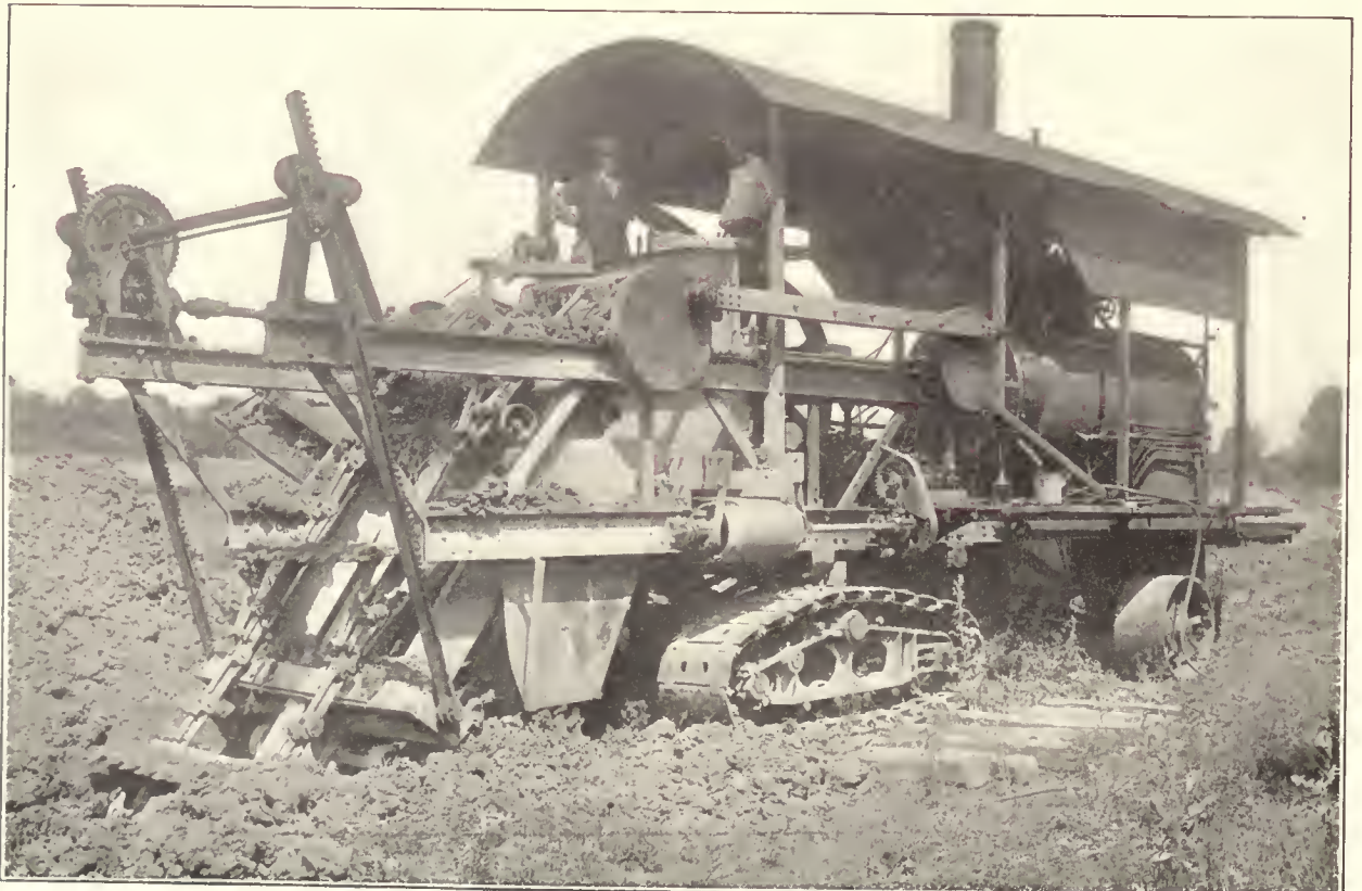
Endless-Chain Bucket Type Trenching Machine with Ladder Racking Gear
