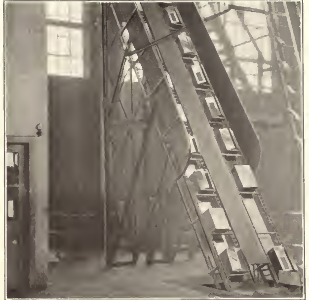
High Angle Double Elevator
