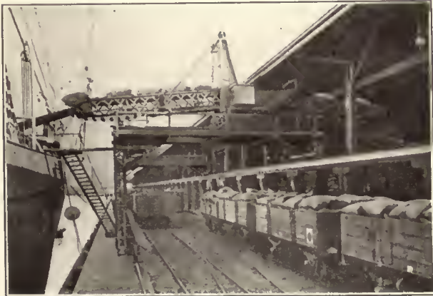
Rapid Loading from Wharf to Ship
