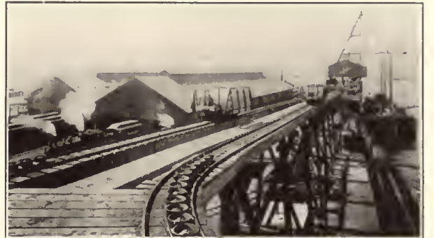
Cable Railway Showing Curves
