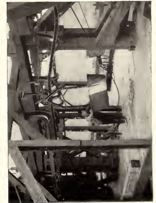
Loading Terminal Showing Carrier with Overhead Grip Passing Down Inclined Rail to Attaching Point
