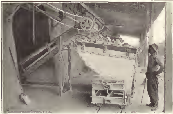
Inclined Bottom Lime Car
