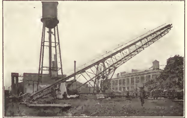
High Piling Saves Storage Space
