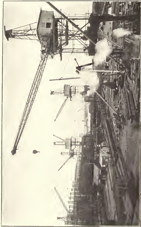
Portal Gantry Cranes Equipped with Boom-Jibs for Shipyard Work
