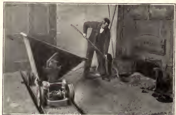
Trunnion Dump Car for Ash Handling
