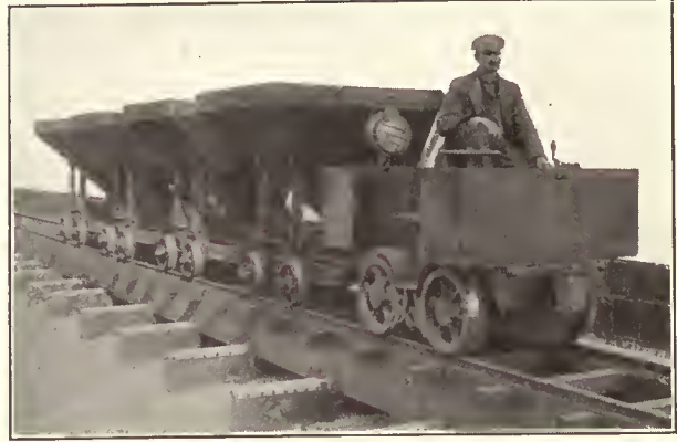
Inclined Bottom, Side Dump, Concrete Cars
