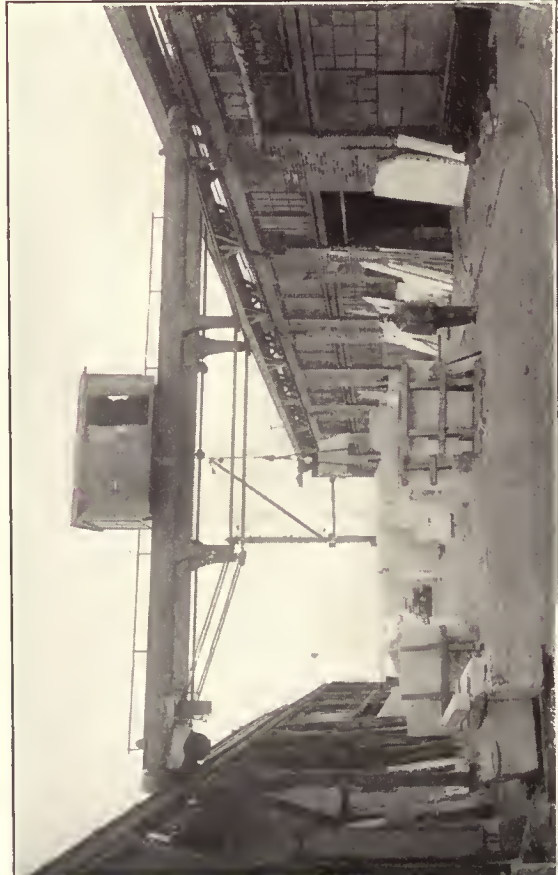
Electric Overhead Traveling Crane Having Truss-rod Type of Bridge and Controlled from Traversing Cab, Handling Stone Slab with Chain Sling
