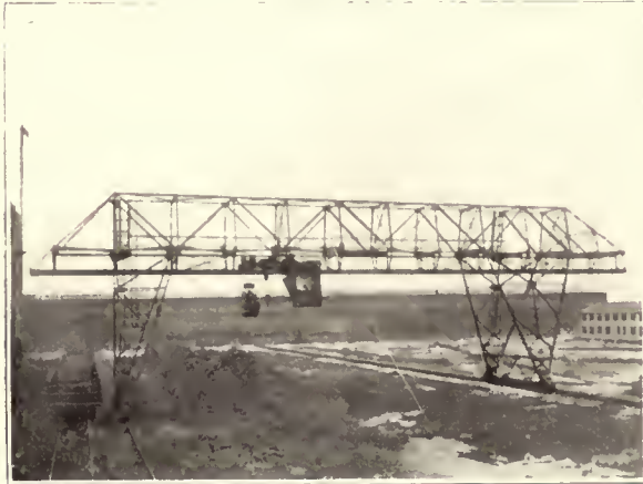
LABRIDE equipped with extra drum and hook. Handles both coal and steel.
