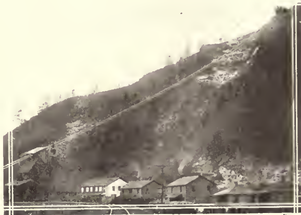
Leschen Single Span Heavy Capacity Two-Bucket Tramway handling coal in West Virginia.
