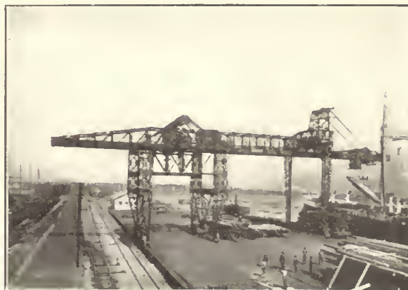
Shaw Wharf Gantry Crane.
