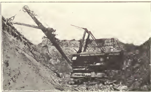
Electric Shovel Digging Power Canal at Niagara Falls, Canada, Operated by A. C. Type MA Motors.
