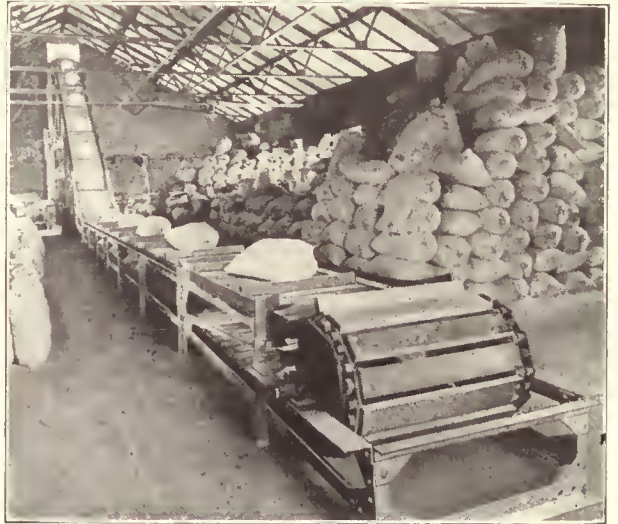
Combined Conveyor and Elevator
