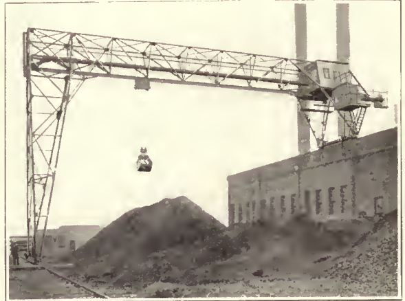
LABRIDE Bridge for Power Plants.
