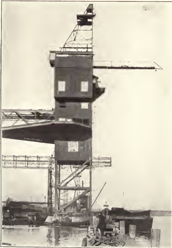
Handling and Cleaning Tower with Conveyor
