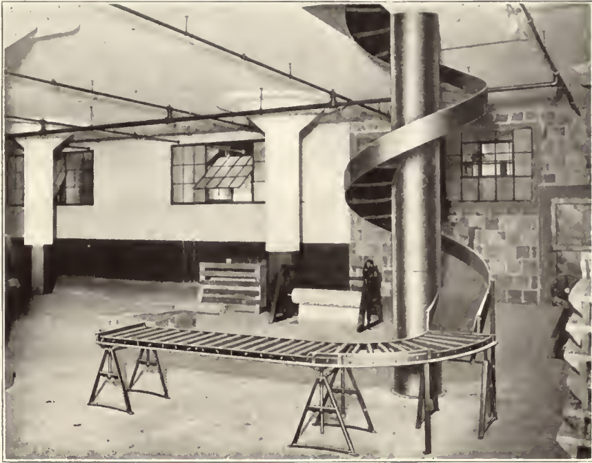
Combination of spiral chute and gravity conveyor.
