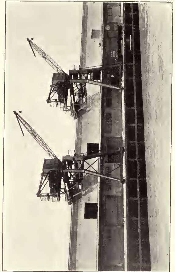
Semi-Portal Wharf Gantry Cranes for Loading or Unloading Cars or Vessels
