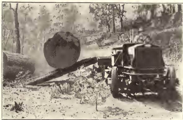
A White 5-Ton truck equipped with White winch and cross-haul loading equipment reduces the loading time in logging from 60 or 70 minutes to as low as 20 minutes.
