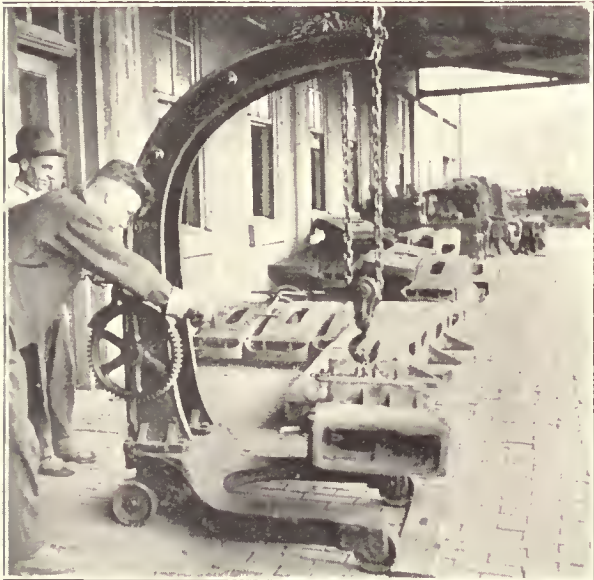
Skeleton-Platform Jib Crane
