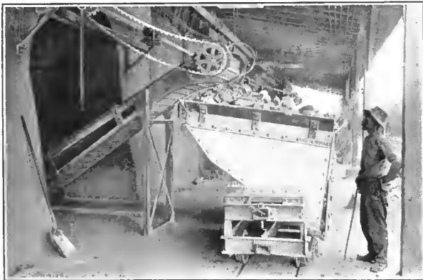
Inclined Bottom Lime Car
