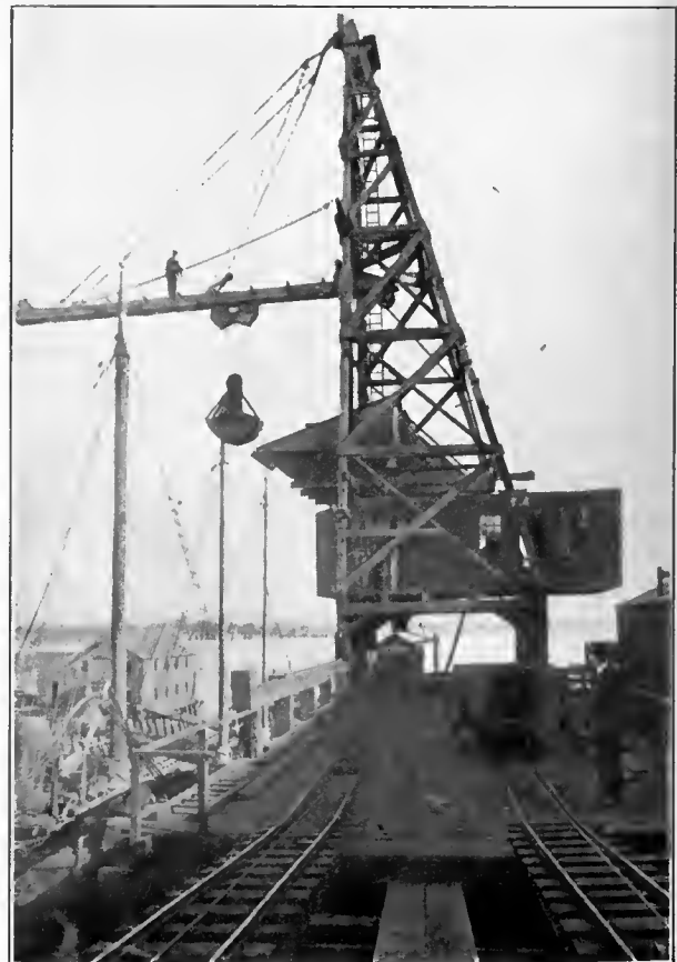
Coal Handling Tower at Power Plant
