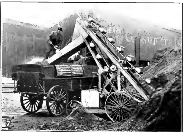
Portable Bucket Loaders: (1) Reclaiming from Storage; (2) Screening and Sizing; (3) Handling Gravel; (4) Car Unloading; (5) Digging and Loading; (6) A Self-Feeder Loading a Truck; (7) Storage to Truck; (8) Radial Type in Construction Work
