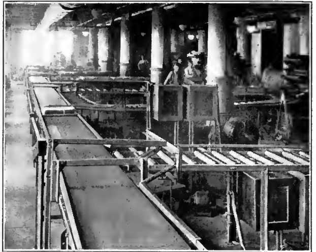
Automatic Selective Switching
