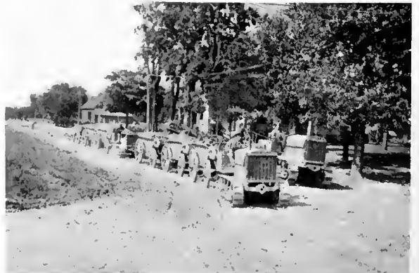
Holt "Caterpillars" replacing 25 horses
