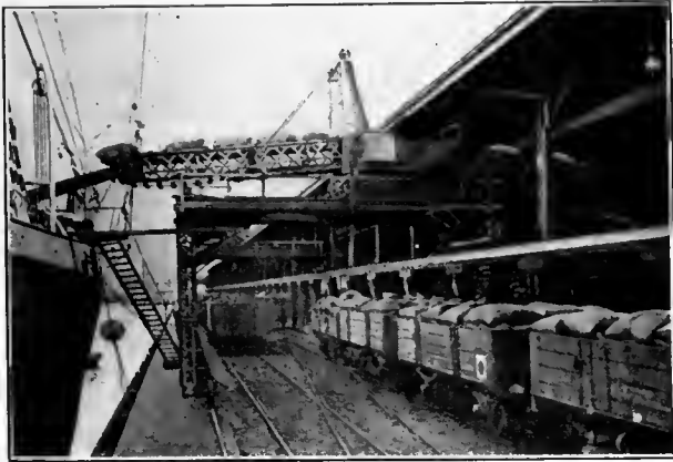
Rapid Loading from Wharf to Ship
