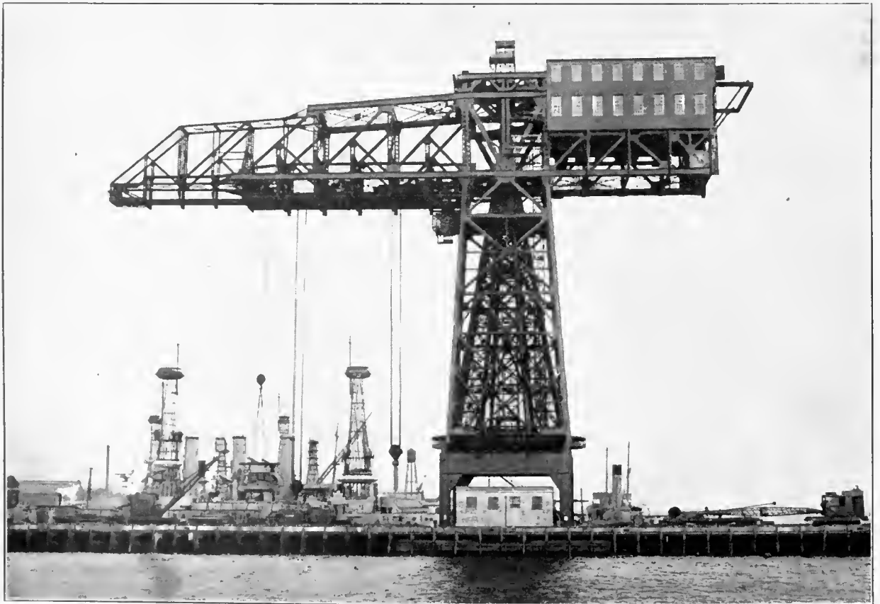
Stationary Hammerhead Portal Crane Installed in Philadelphia Navy Yard. Capacity 350 Tons at 115 ft. Radius; 50 Tons at 90 ft. Radius. Overall Height, 230 ft.
