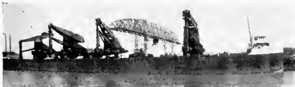
15-Ton Unloaders and Ore Bridge Operated by G-E Equipment.
