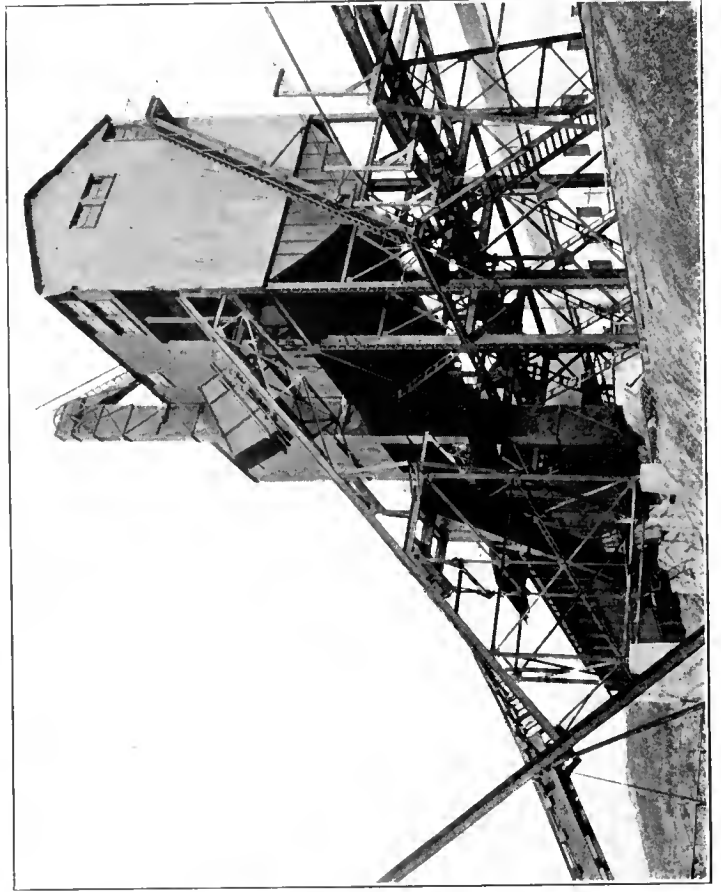
Skip Cars Hauling Coal to Overhead Bunkers
