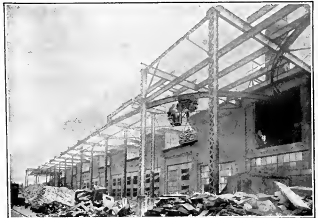
Electric Hoist Cage Control
