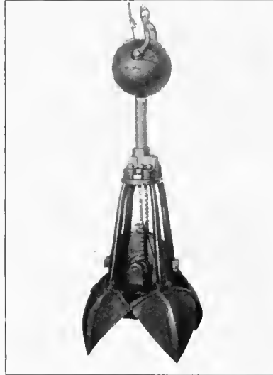
Dwarf Orange-Peel Bucket with Hammer in Raised Position
