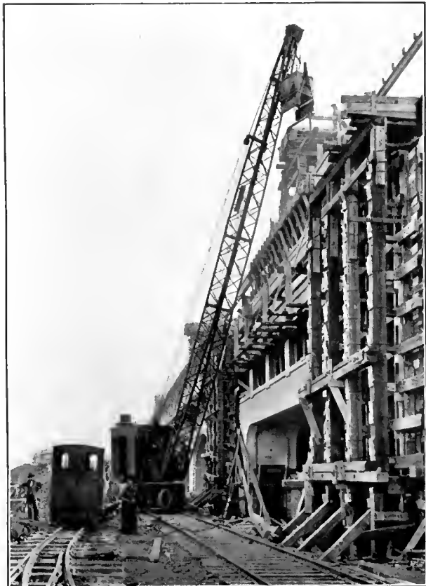
Steam Locomotive Crane Handling Bottom-dump Bucket in Concrete Construction Work
