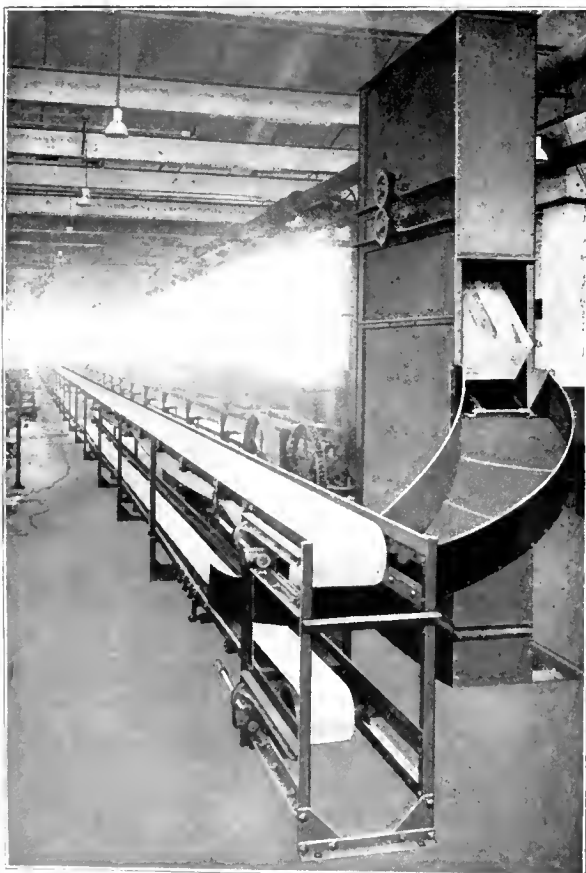
Patented automatic elevator about to discharge to lower run of belt conveyor. Part of American Can Co.'s system, Maywood, Ill.
