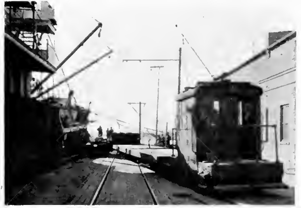
Hauling Material from Ship to Warehouse.
