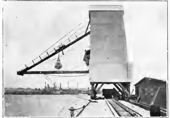
Coal Hoisting Towers.
