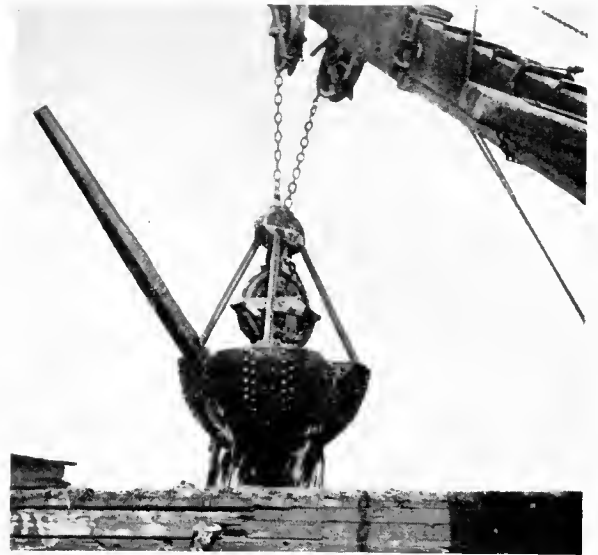
Vulcan Orange-Peel Dredging.
