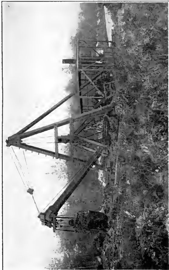
Room Dredge—Barge Derrick—Equipped with Bull-Wheel and Automatic Grab Bucket
