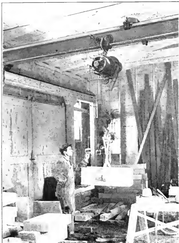
Electric Hoist Installed on Overhead Traveling Crane Handling Block Stone with Stone Tongs
