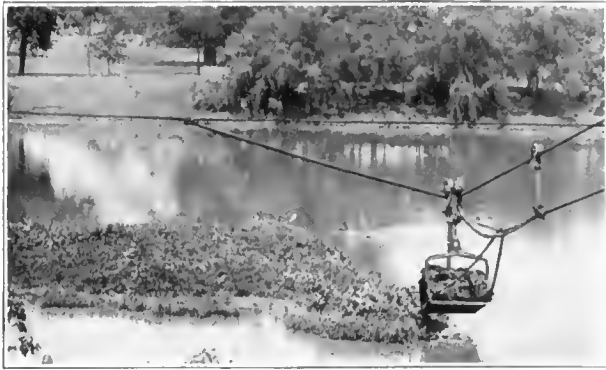
Removing Silt Deposits from Intake Channel.
