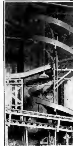
Combination of multiple spiral chute and power driven conveyor.
