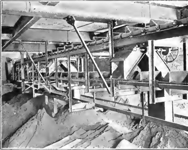
Discharge Chutes on Upper Run
