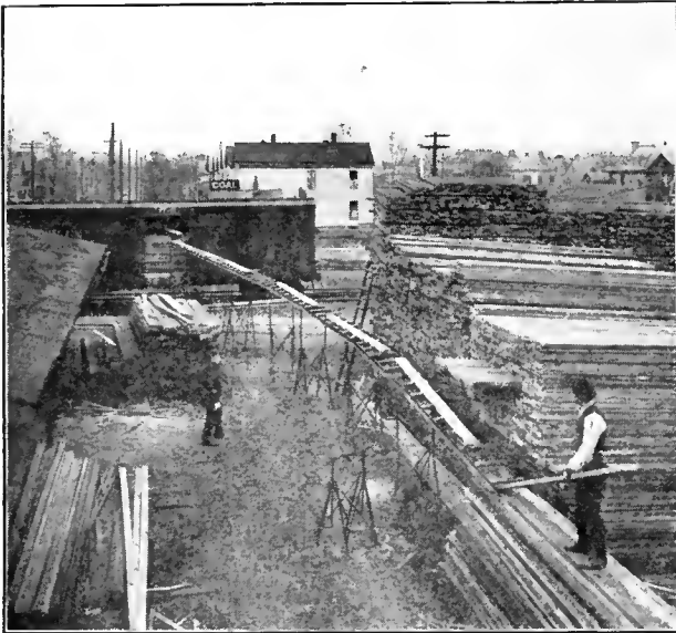
From Car to Lumber Pile
