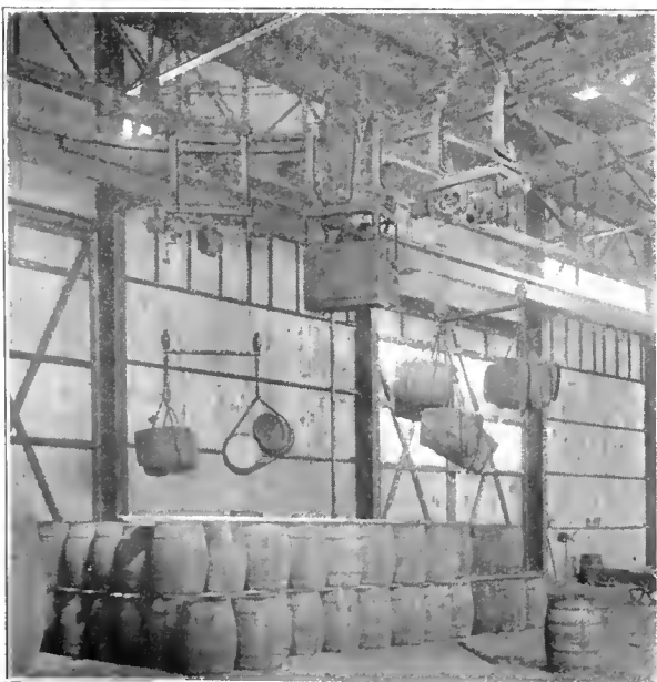
Slings on Spreader Bars
