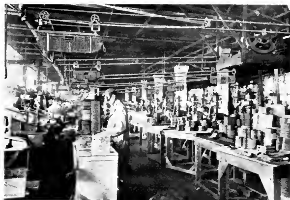
Lamson wire line conveyors in shoe factory carrying dies from die room to operators. They also carry tools, job tickets, time tickets, small parts, laboratory samples, etc. Weimbrenner Co., Milwaukee, Wis.
