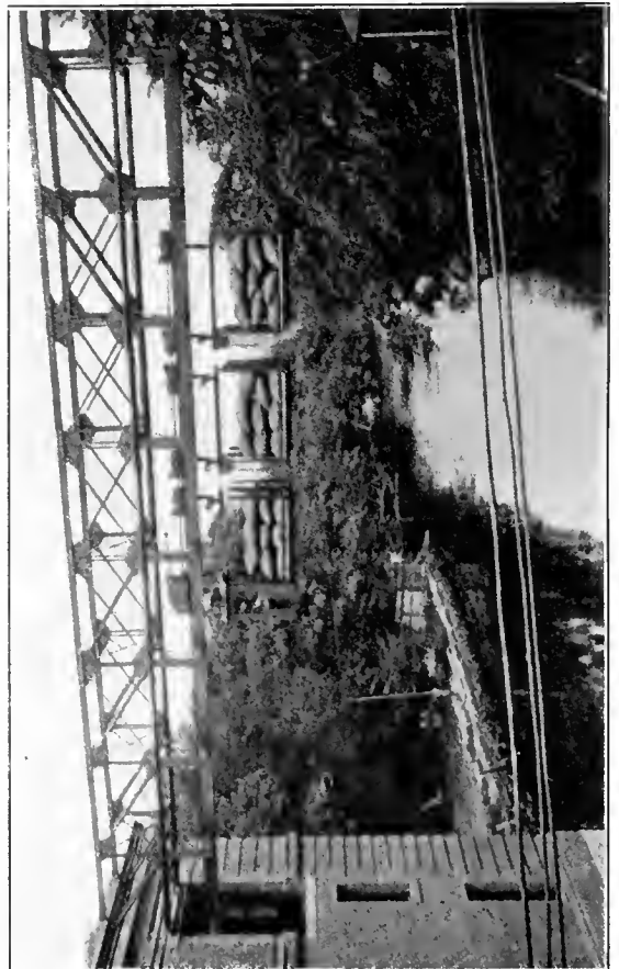
Cab-Operated Monorail Trolley Hauling Trailers Loaded with Bags
