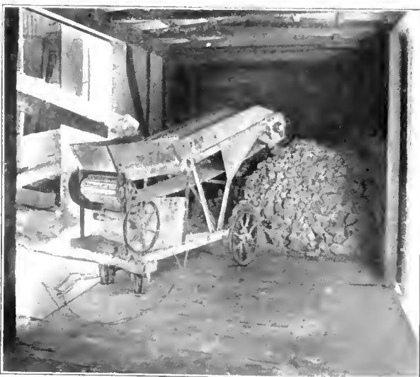
Belt Conveyor Box Car Loader
