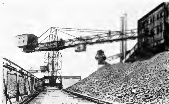
Electrically Operated Gantry Crane Handling Ore.
