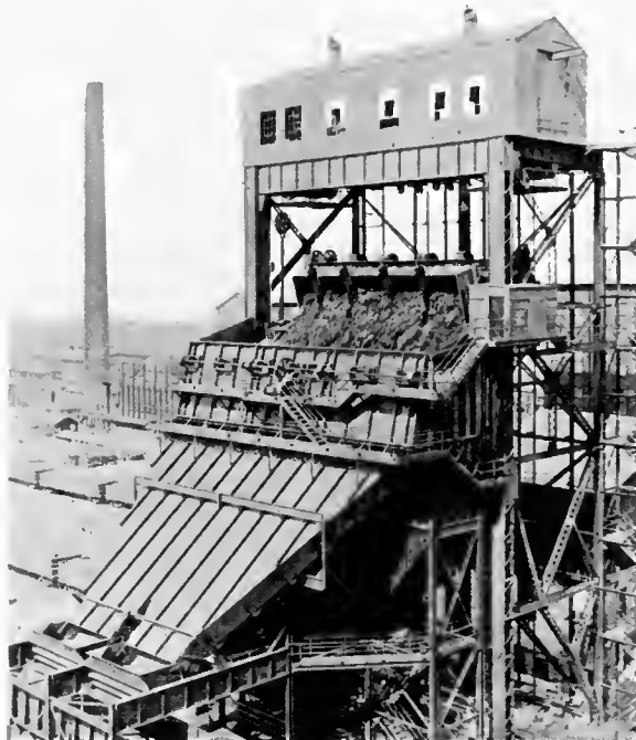
G-E Motors and Control Operating 100-Ton Car Dumper.
