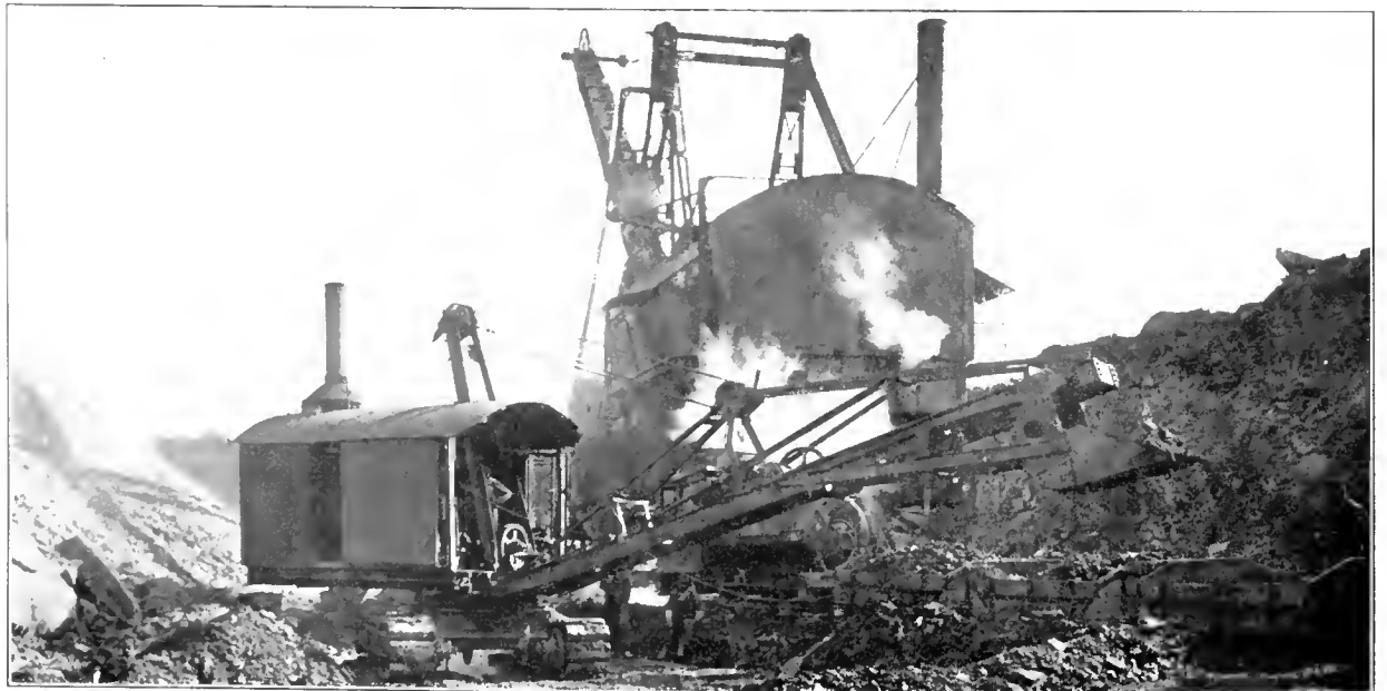
Skimmer or Coal Loader Working in Conjunction with Large Revolving Steam Power Shovel
