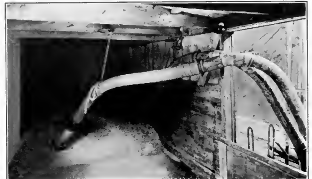
Pneumatic Conveyor Inside a Car
