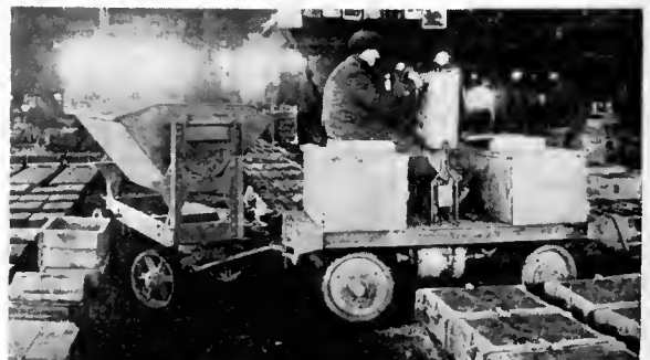
G-E Equipped Electric Tractor Handling Foundry Sand
