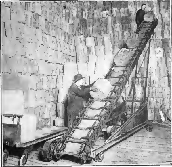
Drop Axle Carrier for Special Packages
