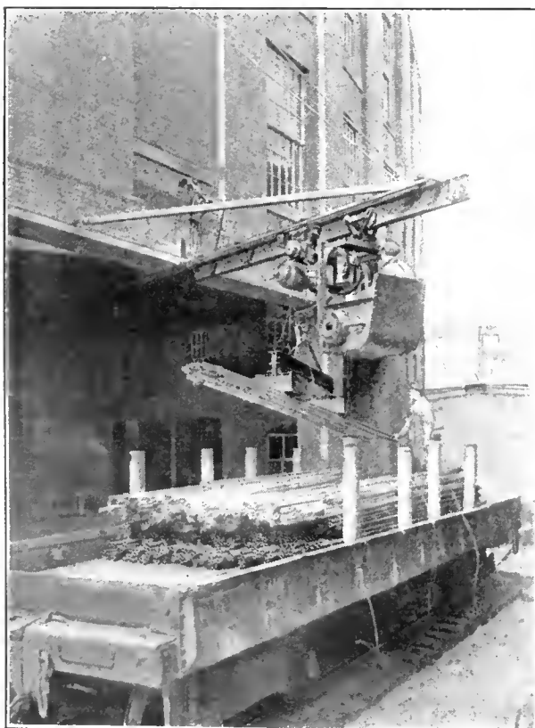
Monorail Hoist Handling Pipe with Rectangular Lifting Magnets on a Spreader Bar
