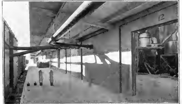
Pneumatic Station for Unloading Grain Cars
