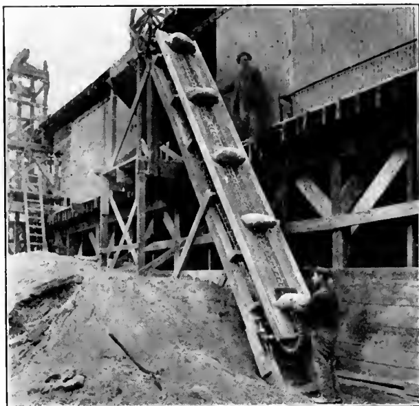
Delivering Cement by Temporary Elevator
