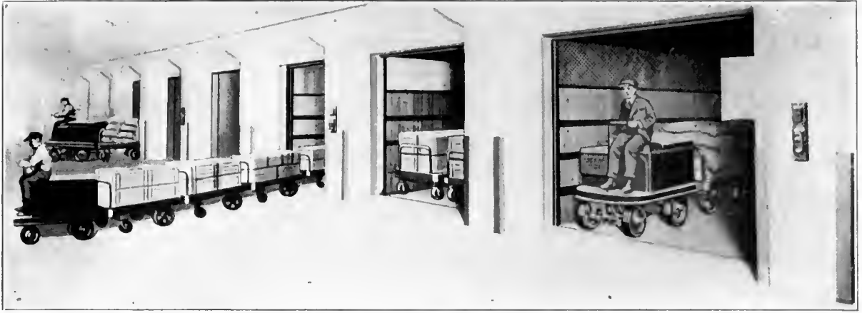
Group of ten Otis Operatorless Elevators in the United States Army Base, showing tractors and trailers unloading from an upper floor.
