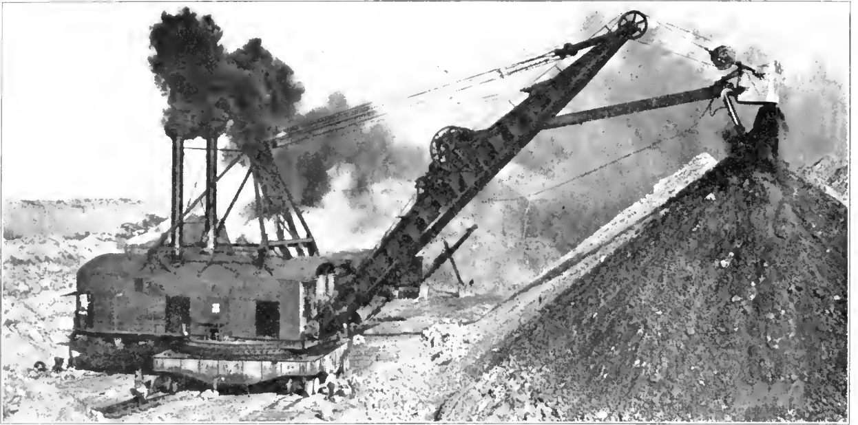
Large Revolving Steam Power Shovel Stripping Overburden in Open Mining Operations
