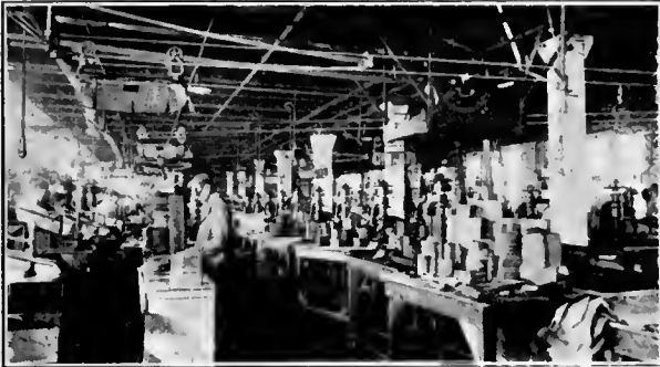
Light Packages Are Distributed Overhead
