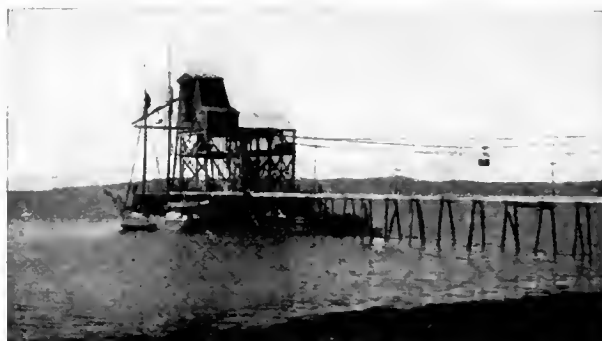
Trenton Aerial Tramway on Dock Haulage Work.
