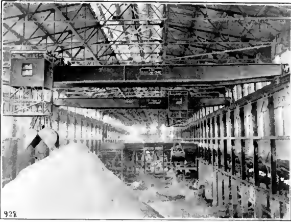
10-Ton Crane Lifting Fertilizer.
