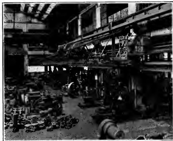
Shaw Wall Crane in Machine Shop.
