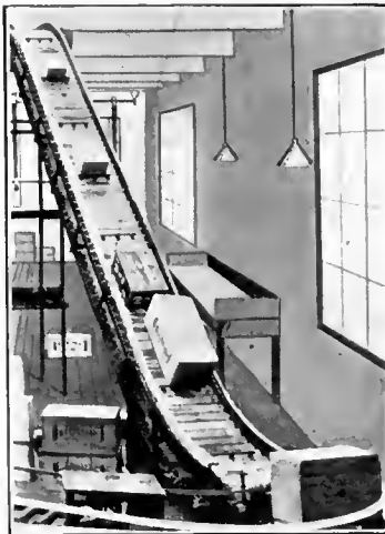
Inclined elevator taking delivery from gravity roller conveyor.
