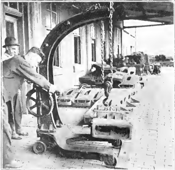
Skeleton-Platform Jib Crane
