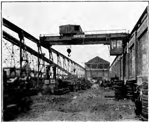
30 Ton Shaw Yard Crane Outside of Shop.
