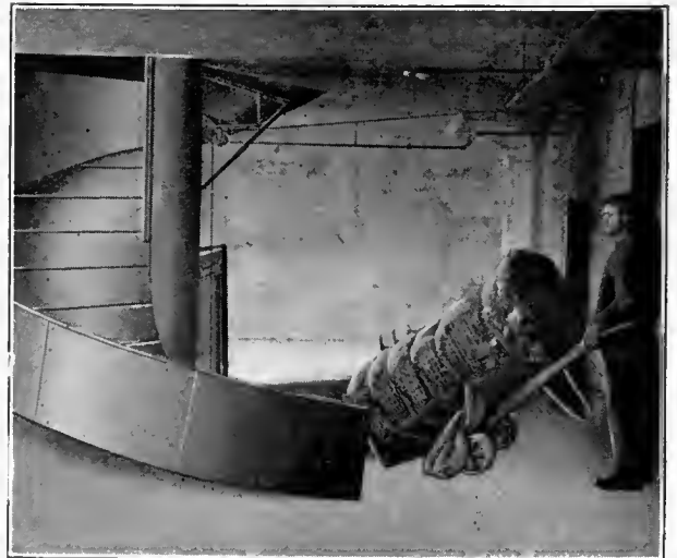
Loading Heavy Bales Through Inlet Gate
