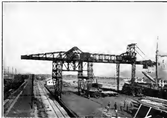
Shaw Wharf Gantry Crane.
