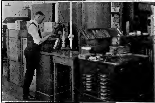
Shop Terminal of Pneumatic Conveyor
