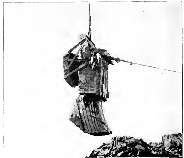
Hinged-Bail Back-Gate Drag-Line Bucket Dumping Soft Clay
