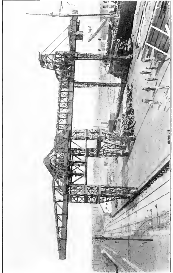
Electrically Operated Double Cantilever Traveling Gantry Crane Designed to Handle Material from Vessel to Storage or to Railroad Cars
