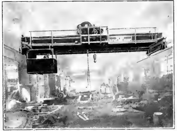
10-Ton Crane in Foundry.
