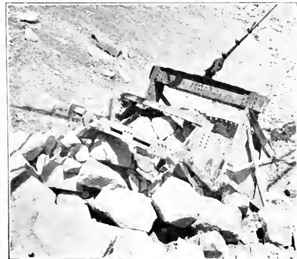
Hinged-Bail Back-Gate Drag-Line Bucket Digging Loose Rock
