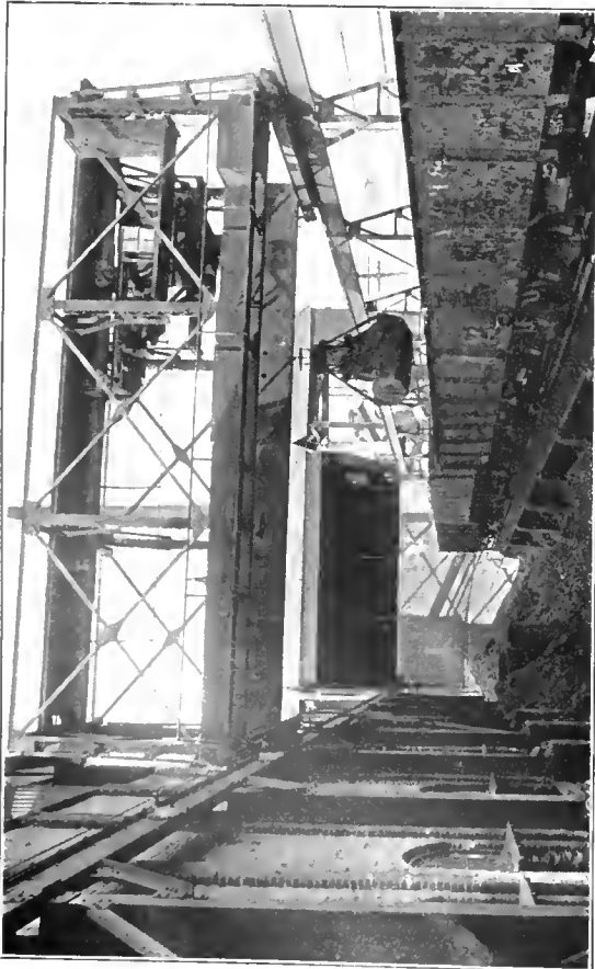
Overhead Traveling Crane Equipped with Automatic Grab Bucket for Handling Coal at a Power House
