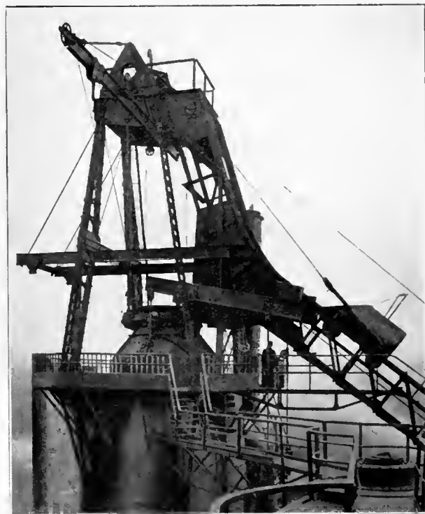
Blast Furnace Skip Car
