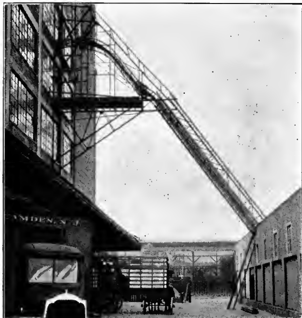
Connecting Operations in Different Buildings
