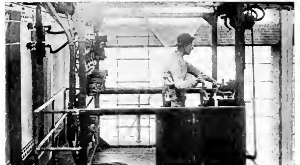
150-Ton Crane Controlled by G-E Magneto Equipment
