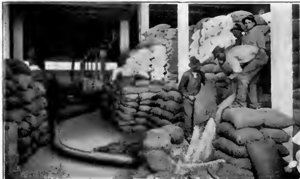
A Warehouse Application
