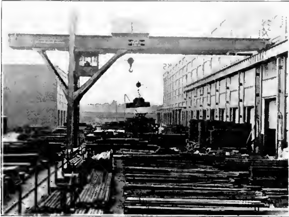
20-Ton Crane in Yard. 1 Leg Gantry.
