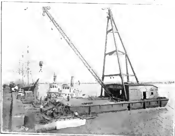
"A" Frame Barge Derricks, 5 to 150 Tons Capacity.
