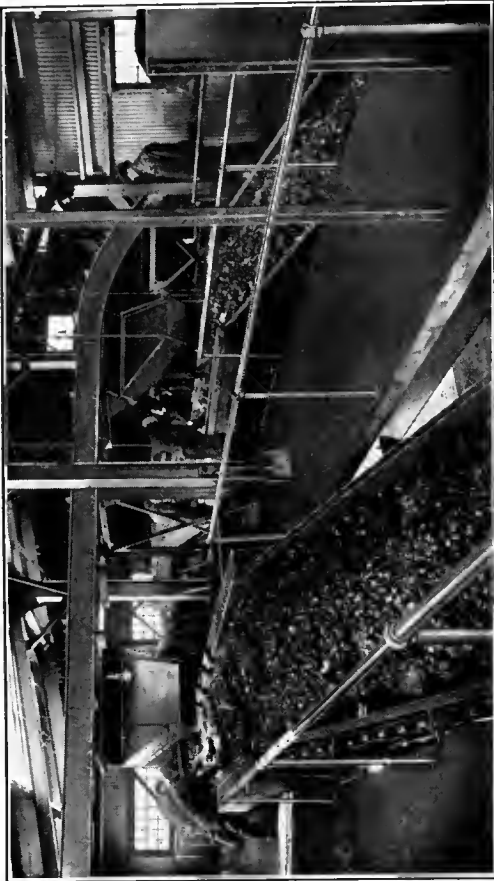
Fig. 10—Picking Table and Loading Boom
