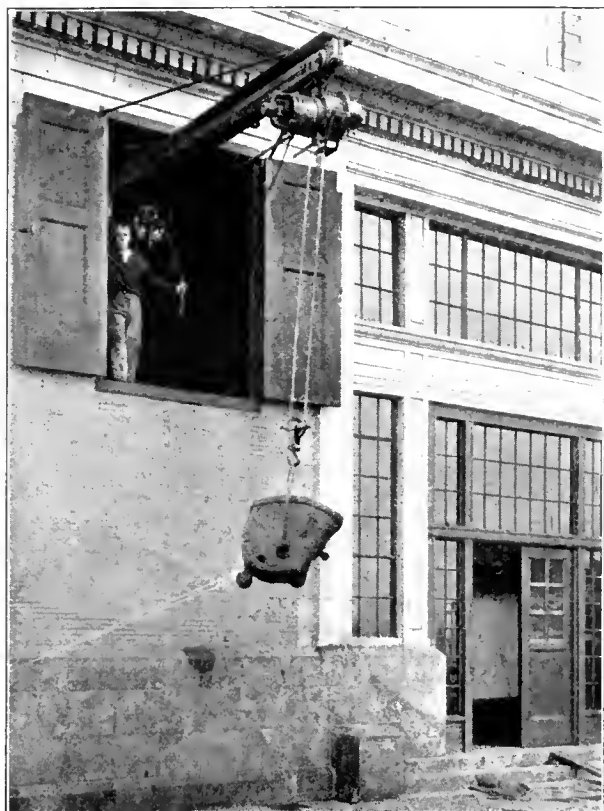
Electric Hoist Installed on Cantilever Monorail, Handling Loose Material with Turnover Bucket
