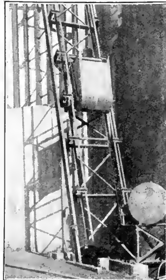
Ash Skip Hoist.
