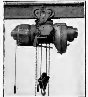
Electric Hoist with Plain Trolley.
