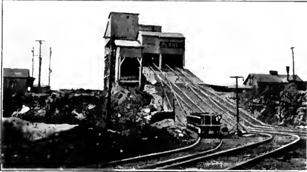
Cable Haulage, Incline
