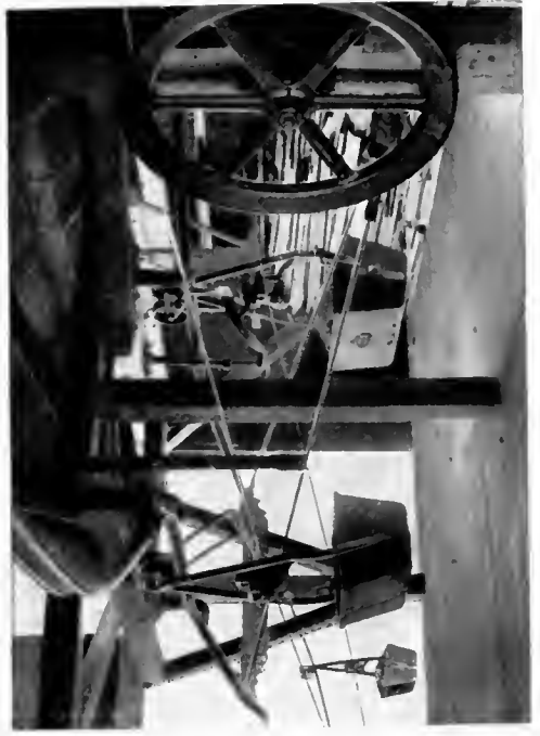
Loading Terminal Showing Carriers with Underhanging Grip in Attaching and Detaching Positions
