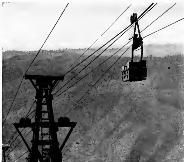
Trenton Aerial Tramway Transporting Slate in Mountains.
