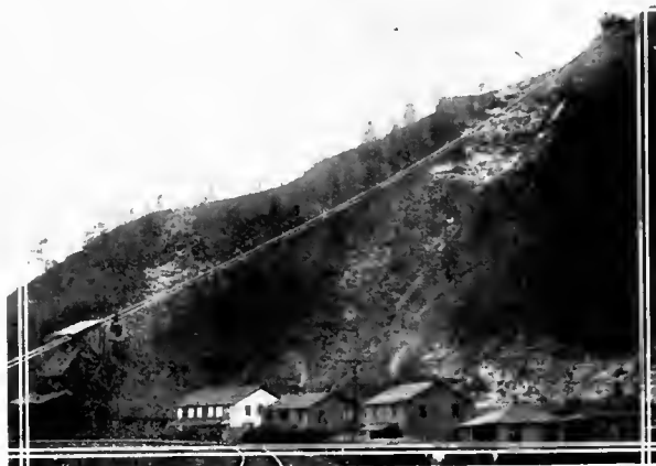
Leschen Single Span Heavy Capacity Two-Bucket Tramway handling coal in West Virginia.
