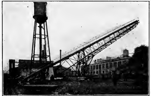
High Piling Saves Storage Space
