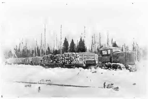
Holt "Caterpillar" keeping the mill running throughout the year
