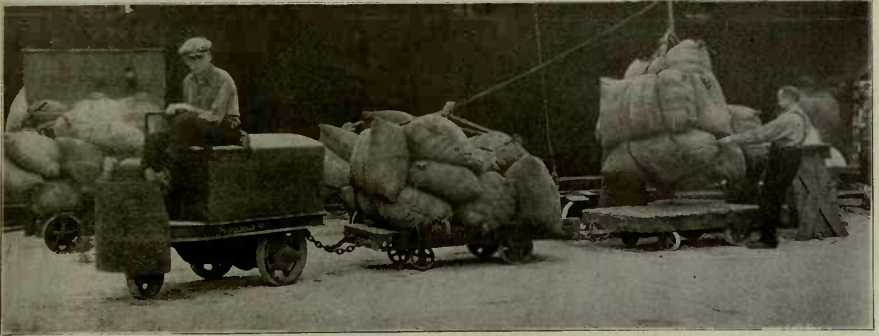
"Trackless Train" moving bagged sugar from ship's side to storage
