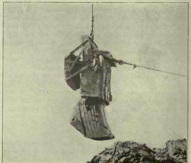
Hinged-Bail Back-Gate Drag-Line Bucket Dumping Soft Clay
