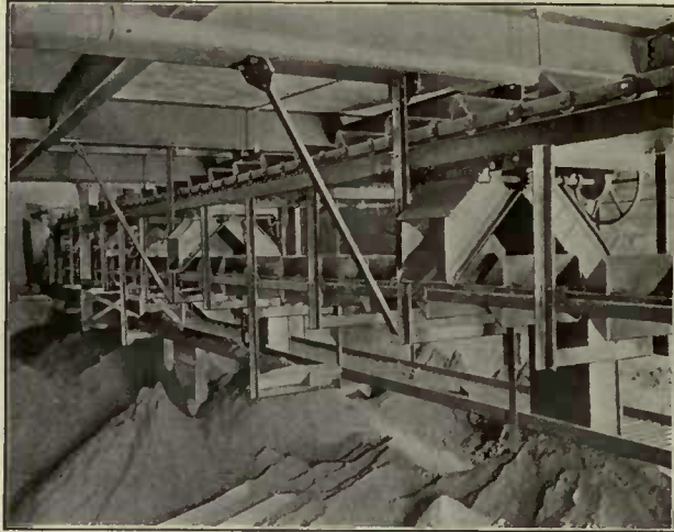
Discharge Chutes on Upper Run
