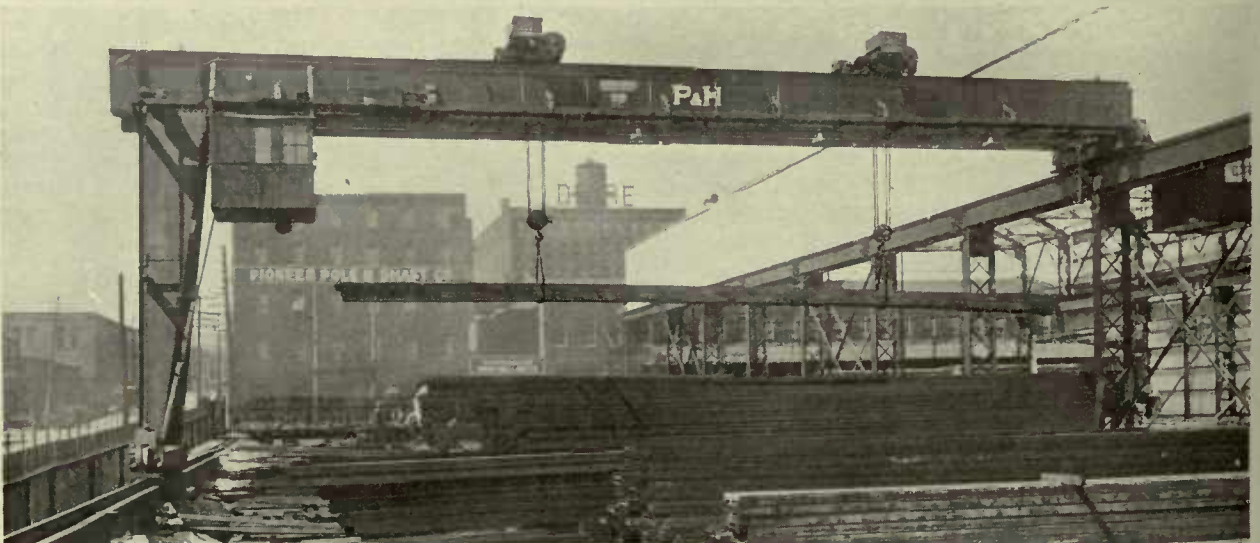
P & H 10-ton single leg double traveling gantry crane handling structural steel material.
