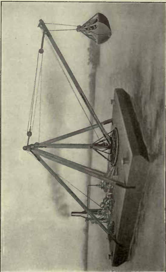
Barge Derrick Equipped with Grab Bucket for Excavation Work or Handling Loose Materials
