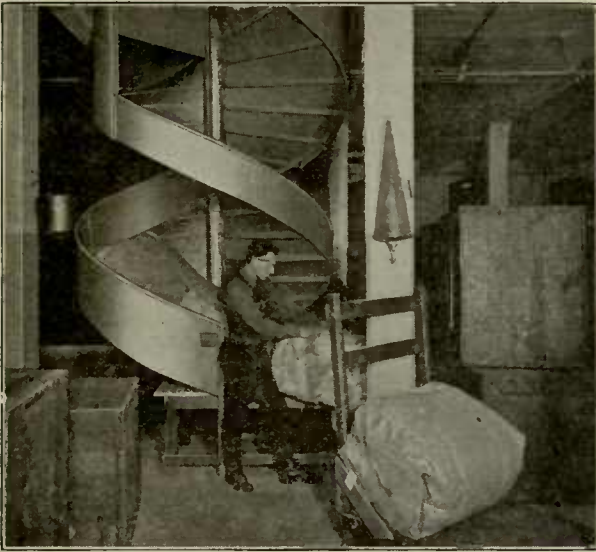
Delivering from Housed Chute to Floor
