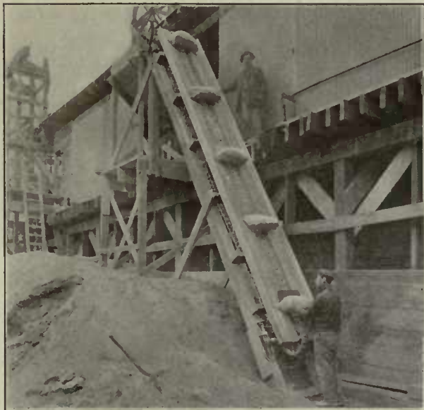
Delivering Cement by Temporary Elevator
