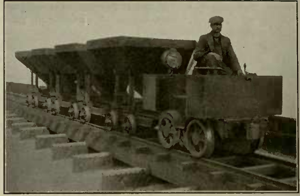
Inclined Bottom, Side Dump, Concrete Cars
