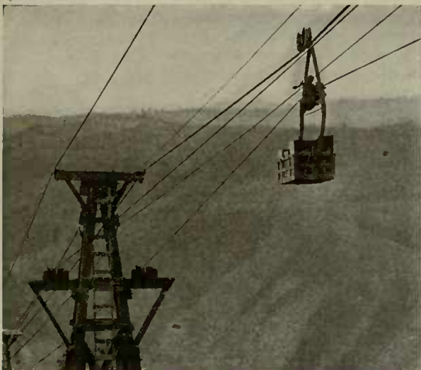
Trenton Aerial Tramway Transporting Slate in Mountains.
