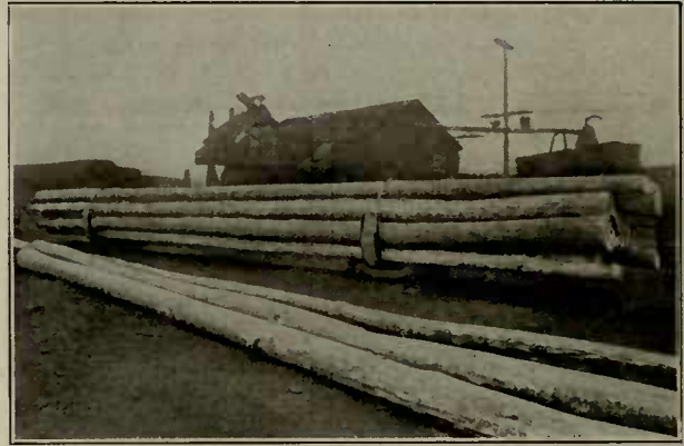
Creosoting Car for Poles
