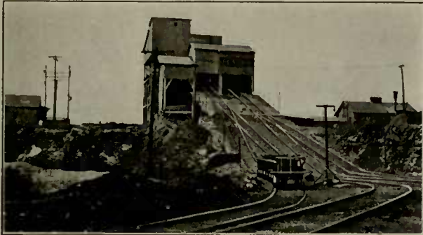
Cable Haulage, Incline
