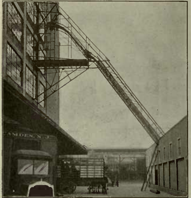
Connecting Operations in Different Buildings
