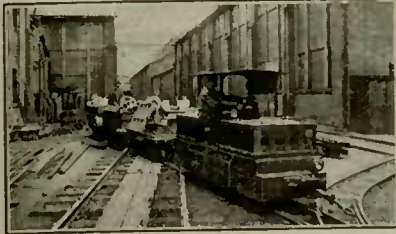
Industrial locomotives equipped with Edison Batteries assure continuous daily service and greater tonnage hauled.
