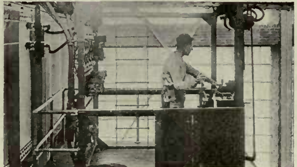
150-Ton Crane Controlled by G-E Magneto Equipment
