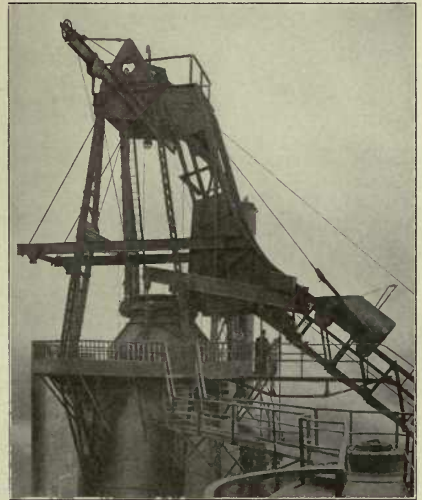
Blast Furnace Skip Car
