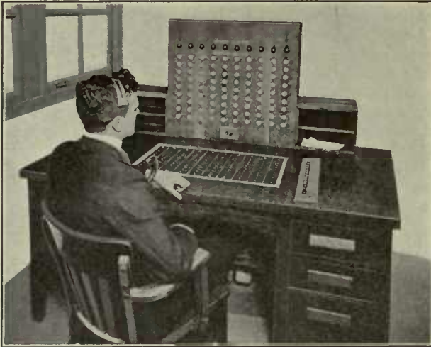
The Dispatcher Controls Ten Elevators
