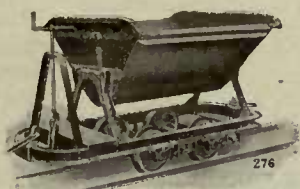
Fig. 276. Standard Cradle Dump Car with Brake.
