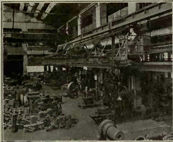
Shaw Wall Crane in Machine Shop.
