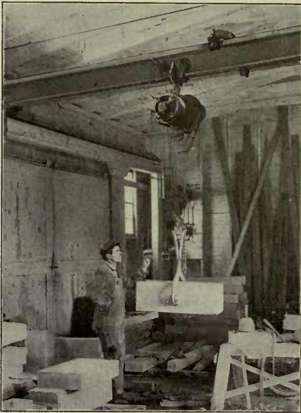
Electric Hoist Installed on Overhead Traveling Crane Handling Block Stone with Stone Tongs
