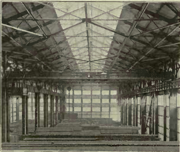
Traveling Crane Handling Steel, Driven by Type K Motors.
