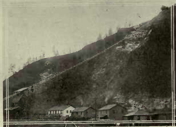
Leschen Single Span Heavy Capacity Two-Bucket Tramway handling coal in West Virginia.
