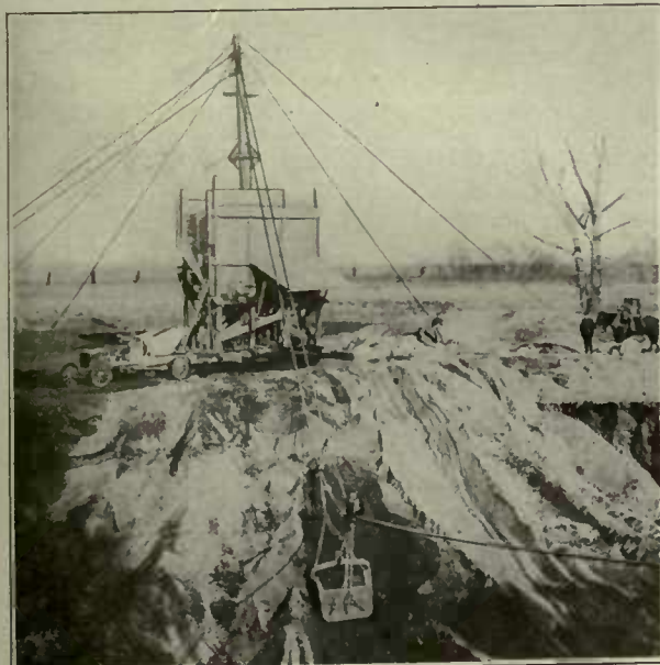
Loading Concrete Aggregate from Pit to Trucks.
