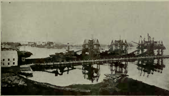
Coal Loading Pier—Machinery Driven and Controlled by G-E Apparatus.
