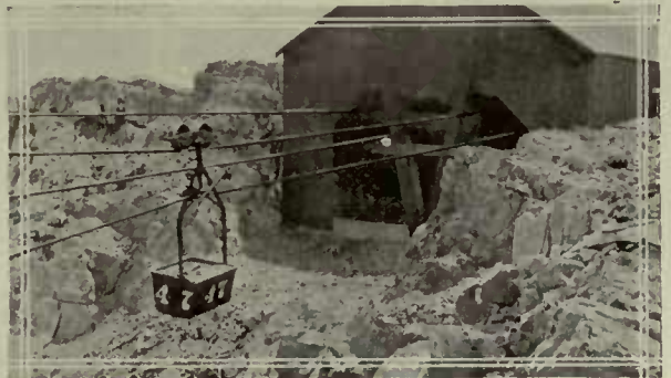
Handling gold and silver ore in the mountains of California with a Leschen Heavy Duty Friction Grip Tramway.
