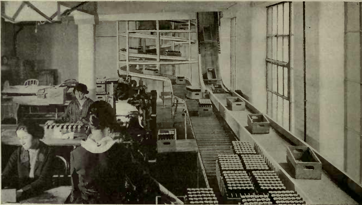
In every Lamson conveyor system the types of conveyors are selected for the particular work they have to do. This picture shows how a Lamson gravity conveyor, spiral conveyor, belt conveyor and booster are combined into one automatic conveying system. Carlton & Hovey Co., Lowell, Mass., Manufacturers of Father John's Medicine.
