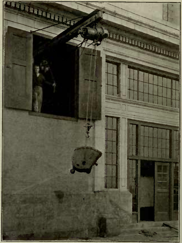
Electric Hoist Installed on Cantilever Monorail, Handling Loose Material with Turnover Bucket
