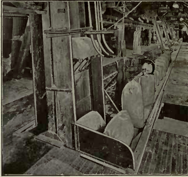
Belt Elevator with Automatic Feed
