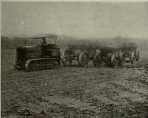
5-ton Holt "Caterpillar" hauling plant refuse
