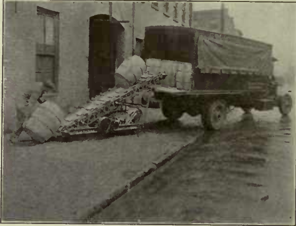
Standard Type Piler with Drop Axles Loading Barrels Into a Truck.
