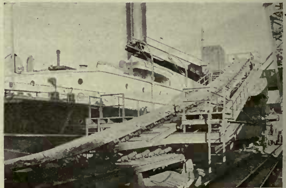
Electrically Operated Belt Conveyor and Loading Boom at Coaling Pier.
