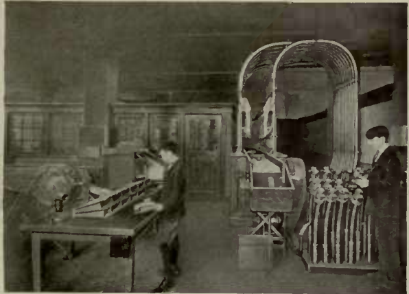
This Lamson pneumatic tube system transmits orders in a few seconds to any department in the large wholesale warehouse of Lehn & Fink, Inc., New York.
