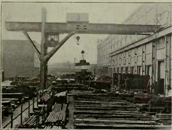
20-Ton Crane in Yard. 1 Leg Gantry.
