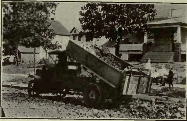
In road building work White trucks with dump bodies handle economically any sort of road materials.
