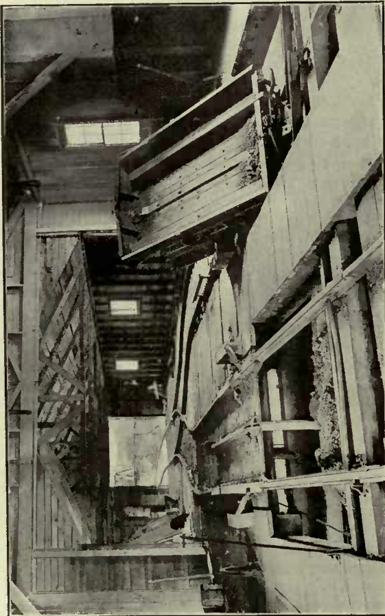
Fig. 1. Cross-Over Car Dump
