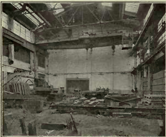
60 Ton Shaw Crane in Foundry.
