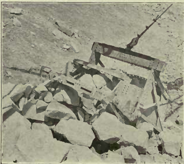
Hinged-Bail Back-Gate Drag-Line Bucket Digging Loose Rock
