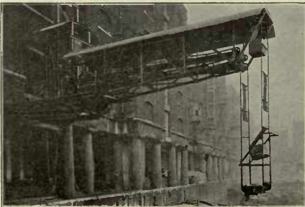
Cantilever Type Sling Conveyor
