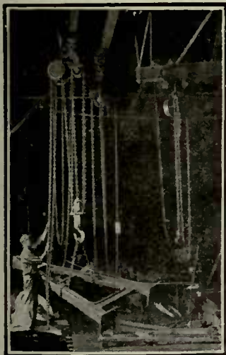
This Foundry's Right Arm. The Wright High-Speed Hoist.
