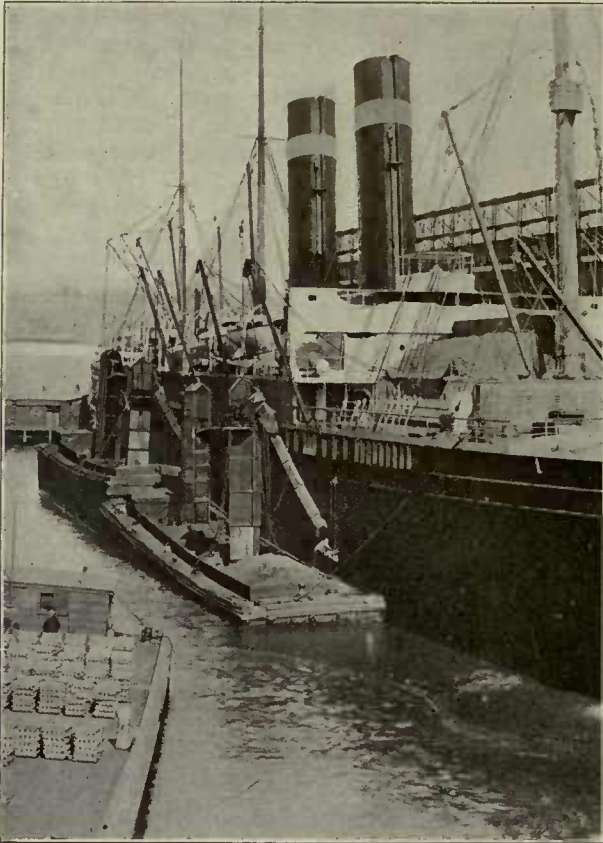
The Discharge Is Through Telescopic Chutes
