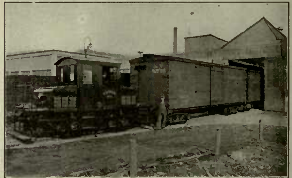
B-W Storage Battery Locomotive in the Plant of Victor Talking Machine Co.
