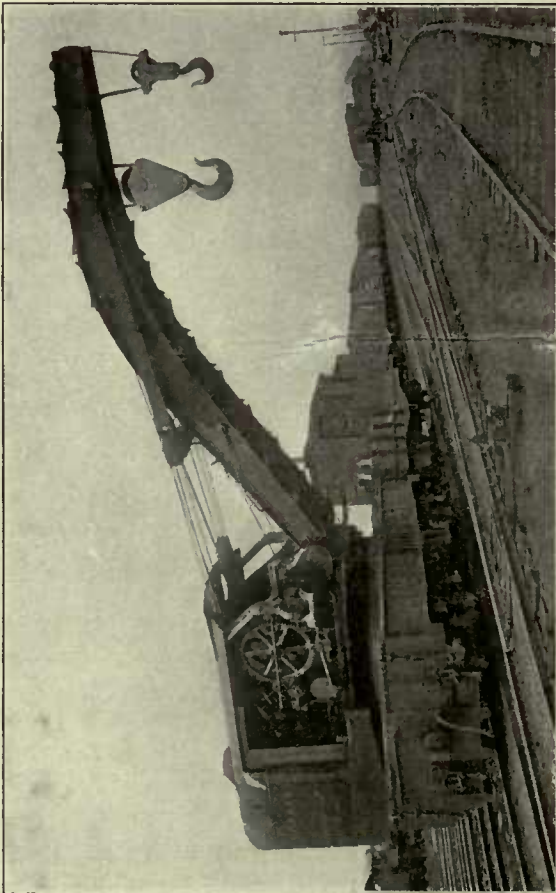
Steam Locomotive Wrecking Crane with Auxiliary Car. Boom Extended to Maximum Radius.
