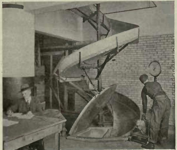
This Lamson spiral chute carries products from a number of floors to a delivery point on first floor. Note hinged fire door which also serves as deflector when goods are delivered at intermediate floors. Army Base Warehouse, Boston, Mass.
