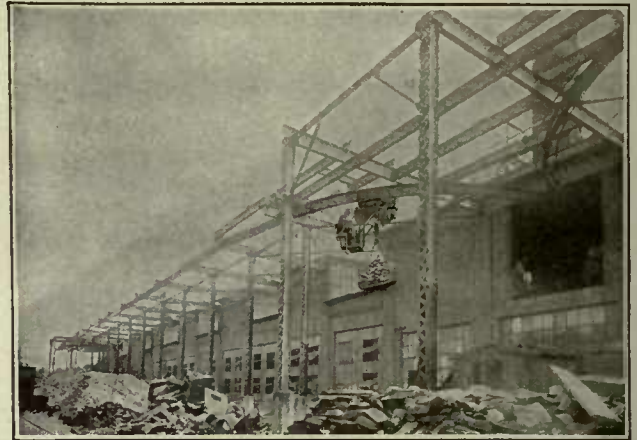
Electric Hoist Cage Control
