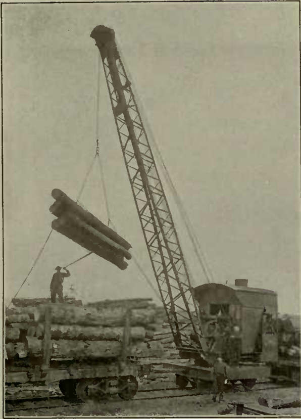
Four-wheel Steam Locomotive Crane Handling Logs with Grab Hook and Chain Slings
