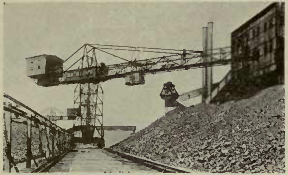
Electrically Operated Gantry Crane Handling Ore.
