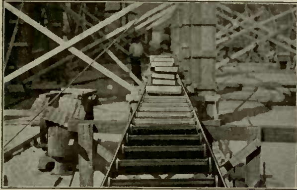
Roller Gravity Convenient in Construction
