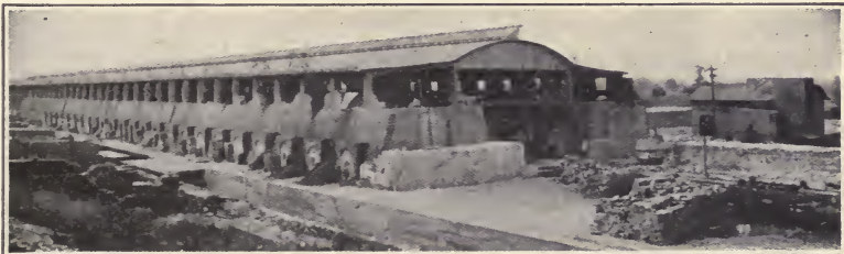
FIG. 56.—Hundred and ten chamber Haigh continuous kiln. Five fires. ( American Clay Machinery Co. )
