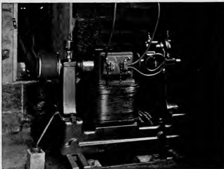
DYNAMO SUPPLYING ELECTRICITY TO THE PHYSIC LECTURE HALL.
