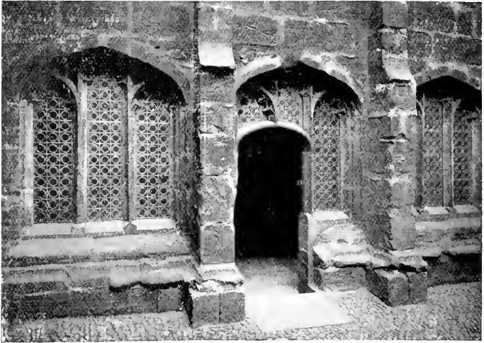
WEST SIDE OF THE CLOISTER.
