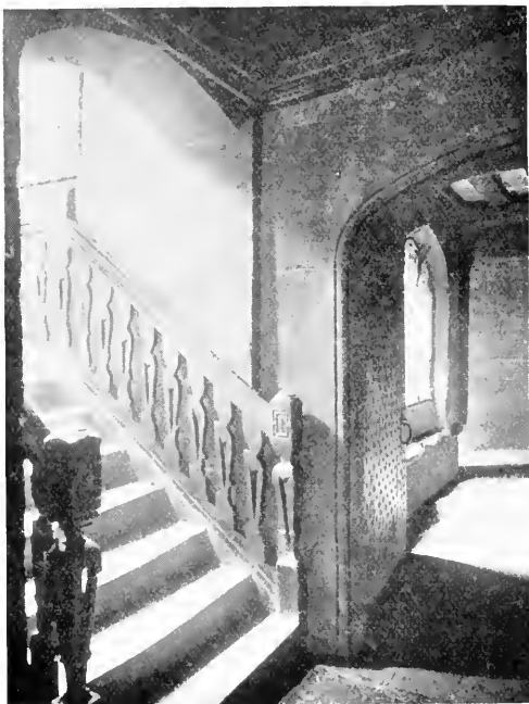
STAIRCASE LEADING TO CLOISTER GALLERY.
