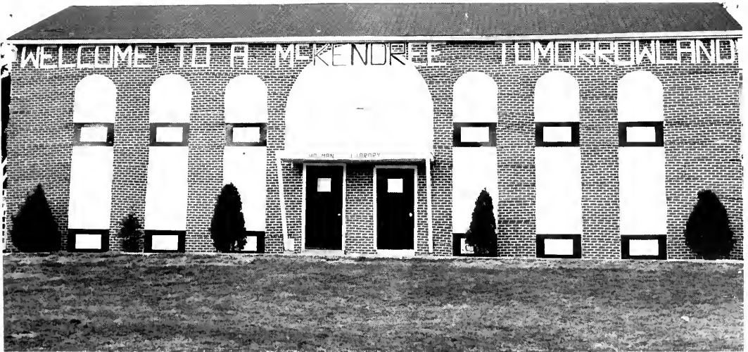
The Ferox Construction Company erects Holman Library in record breaking time to take 2nd place.
