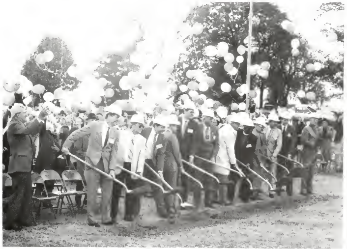
Groundbreaking for the new Convocation Center.
