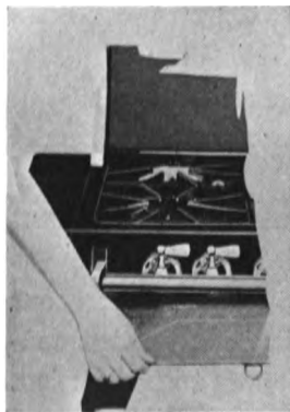
FIG. 4. Part of gas stove showing air mixers.
