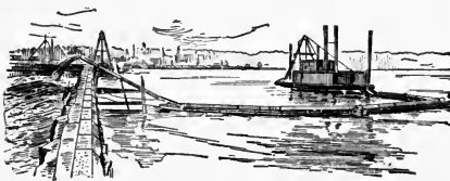
1259. MARINE DREDGE, discharging on the shore through a long floating pipe. Pipe buoyed by pontoons. For harbor work.
