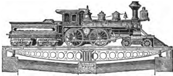
1507. IRON FRAME TURN-TABLE, showing design of cast-iron panels. Wrought-iron top chord.
