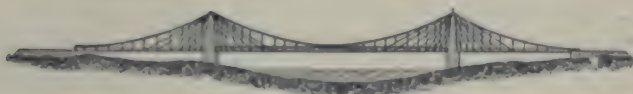
1508. SUSPENSION BRIDGE.—The Cincinnati bridge, "Roebing" system. Ten hundred and fifty-seven feet between piers.
