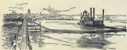
1259. MARINE DREDGE, discharging on the shore through a long floating pipe. Pipe buoyed by pontoons. For harbor work.
