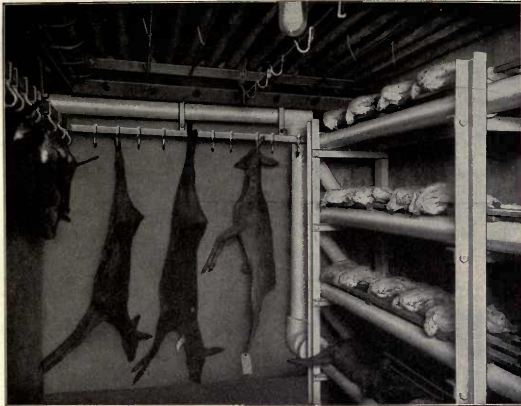
Fig. 9 Cold Storage Room
