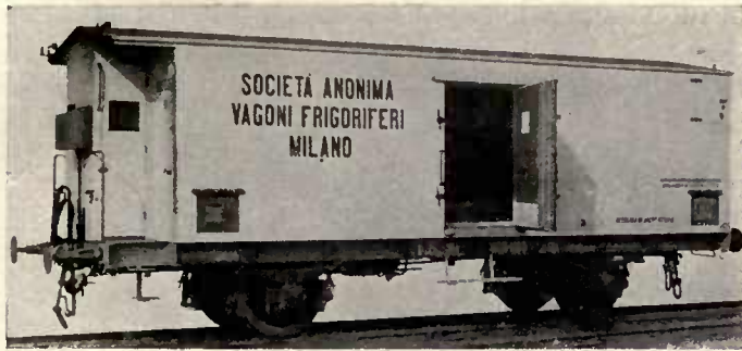
Fig. 5 Refrigerator Van insulated with Expansit Cork Stone
