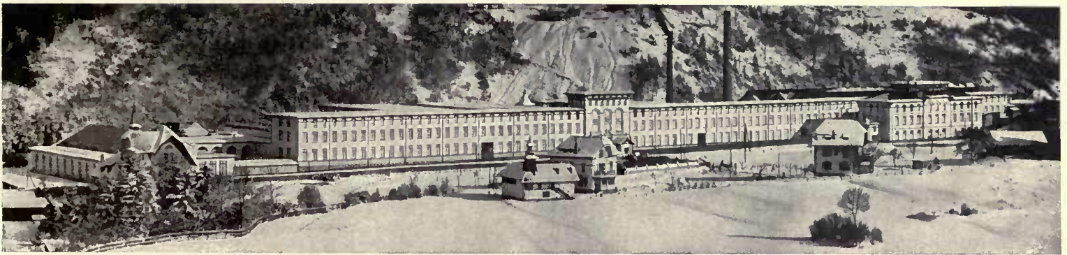
Fig. 6 Cailler's Chocolate Factory, Broc (Switzerland). Insulated Area about 85 000 sq. ft.
