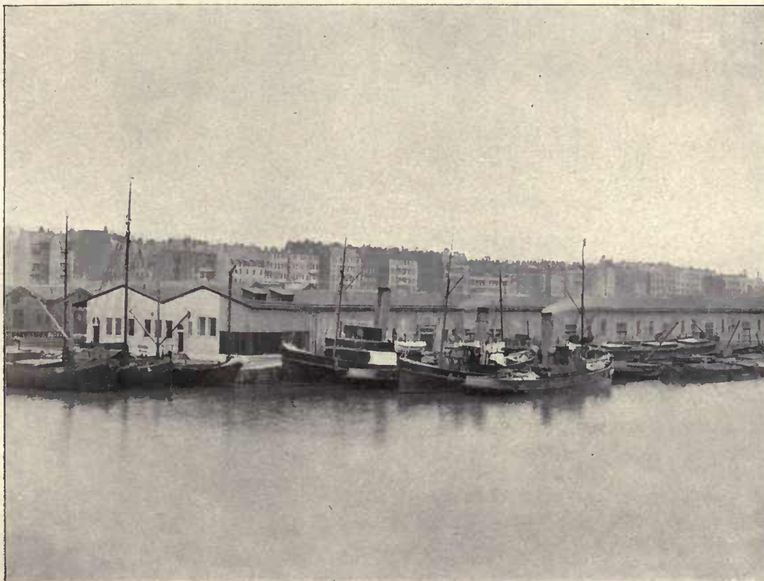
Fig. 5 View from the Harbour
