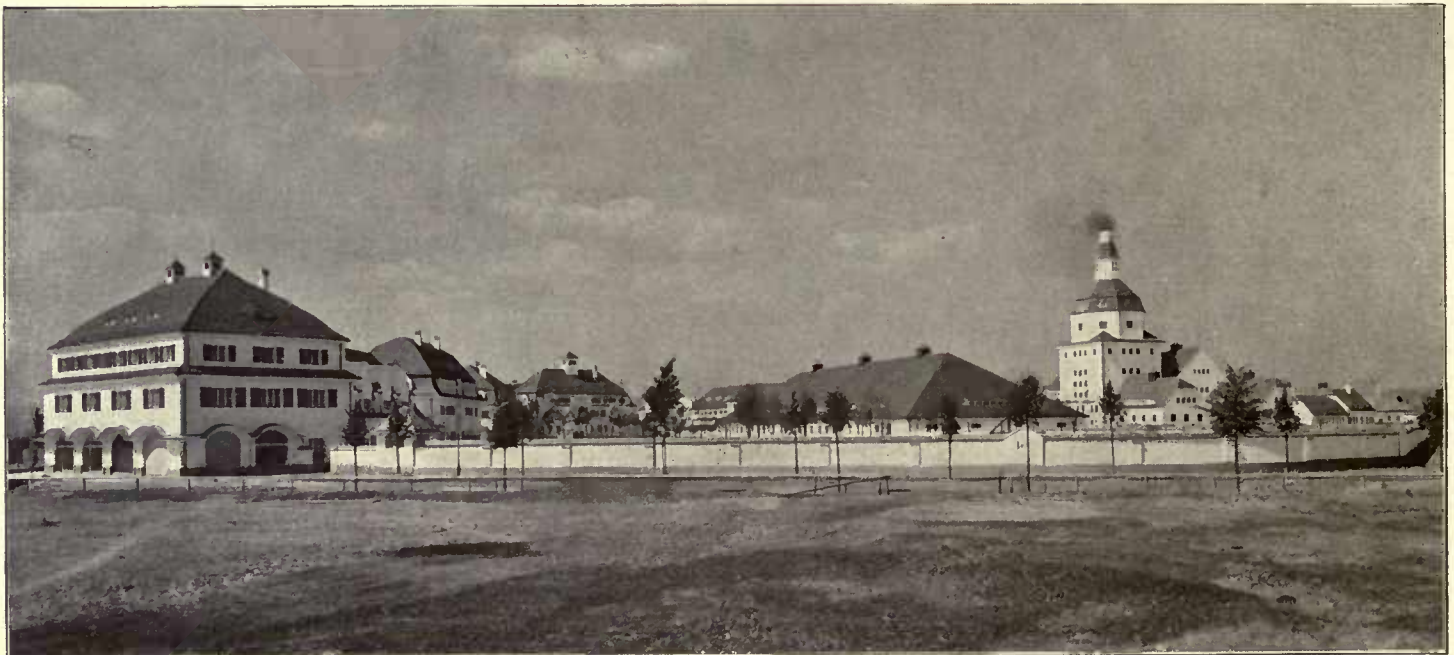
Fig. 10 View from the Abattoir Street
