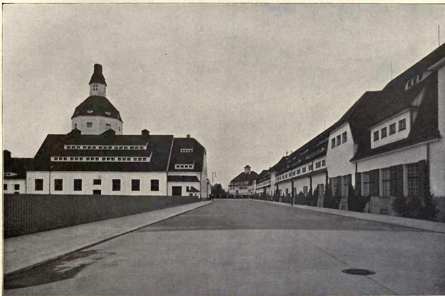
Fig. 6 Road through the Abattoir
