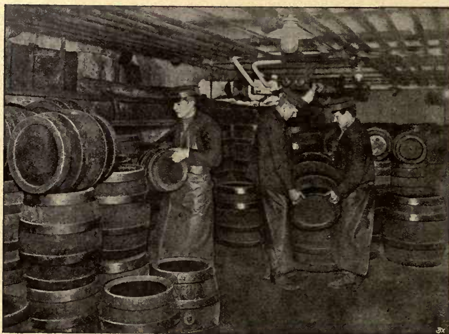
Fig. 18 Beer Cold Storage Room
