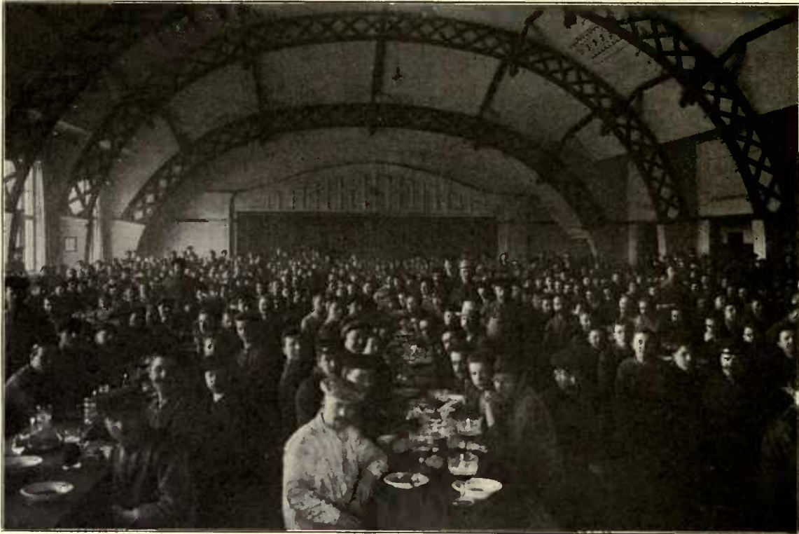
Fig. 13 Dining Hall for Workmen
