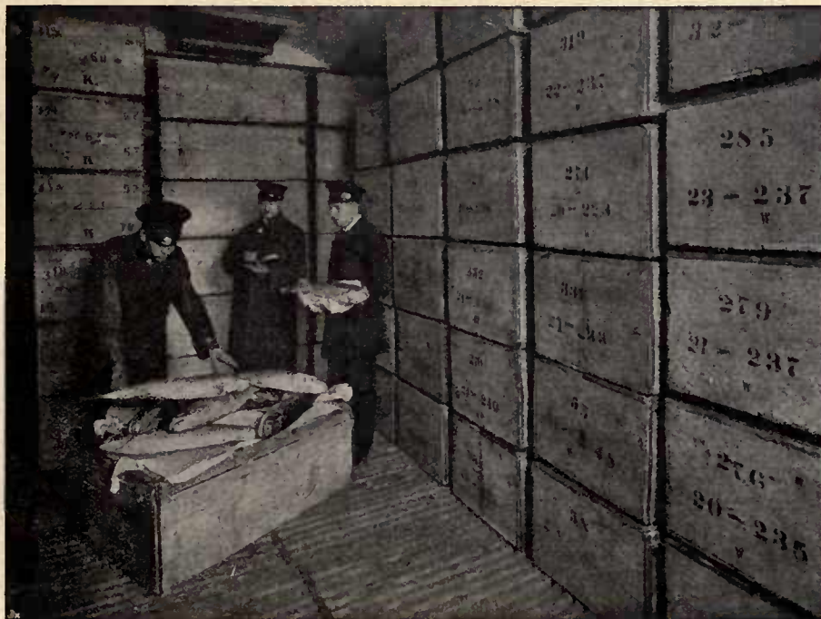
Fig. 16 Fish Cold Storage Room
