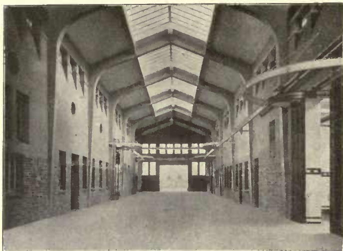
Fig. 2 Communication and Traffic Hall
