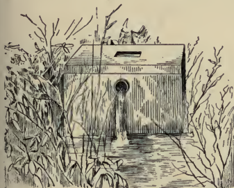
FIG. 126.—Concrete cover for a spring.
