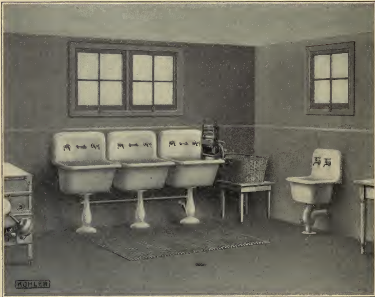
FIG. 83.—Enamel wash trays in a basement laundry.
