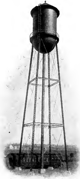
Fig. 90. A modern form of water-tank. (Erected at St. Elmo, Ill., by the Chicago Bridge and Iron Works.)
