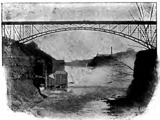
Fig. 77. The Driving Park Bridge at Rochester, N. Y.
