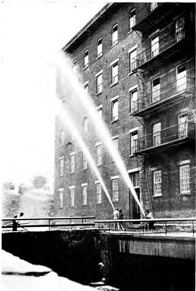
Force illustrated by two fire streams being delivered by the pump service of the large cotton mills of B.B. & R. Knight at Natick, Rhode Island. One stream is being held by men in correct position, the other by men who have been crowded into an awkward and dangerous position. Pressure shown on the gauge at the hydrant was 75 pounds per square inch.
