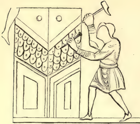
TILING WITH WOODEN SHINGLES.
