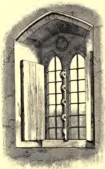
UNGLAZED WINDOW AT COGGS.
