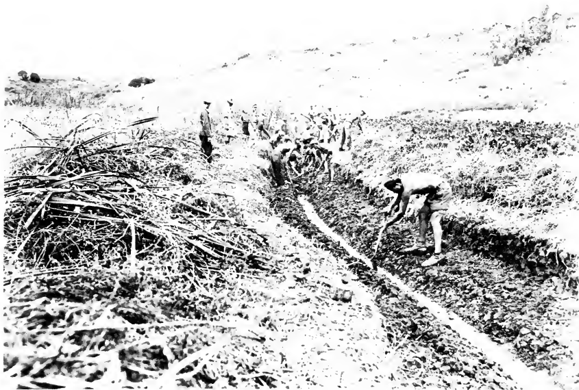
ITALIAN POW'S DRAINING SWAMPY GROUND near Algiers as a malaria control measure.
