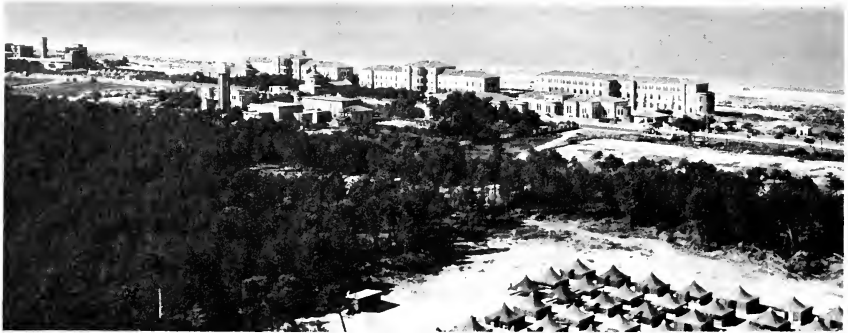
12TH GENERAL HOSPITAL, the largest unit in the group of medical installations in the northern outskirts of Leghorn.
