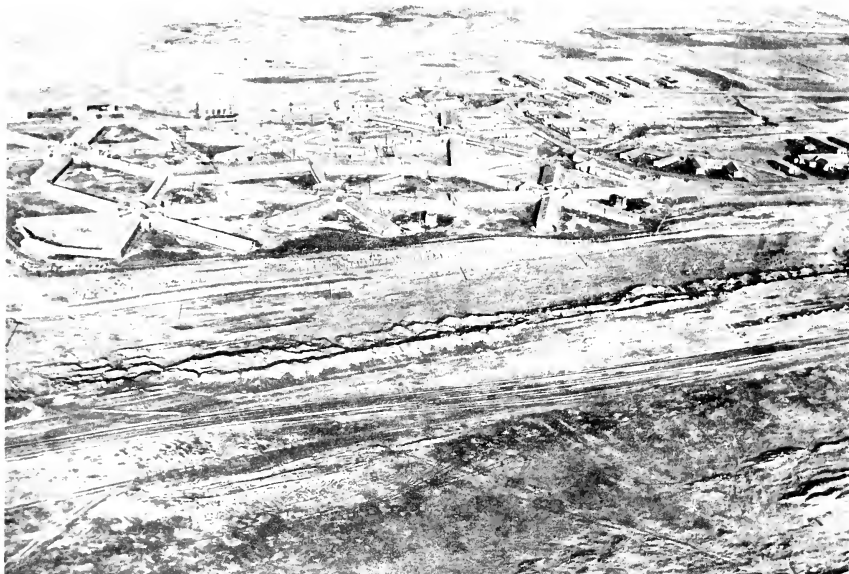
113TH GENERAL HOSPITAL AT AHWAZ, IRAN, laid out in radial pattern with connecting wings.
