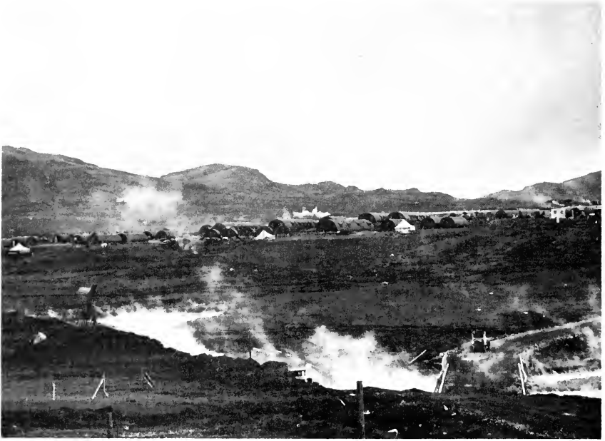
167TH STATION HOSPITAL at Alafoss, Iceland, showing hot springs used to heat buildings.
