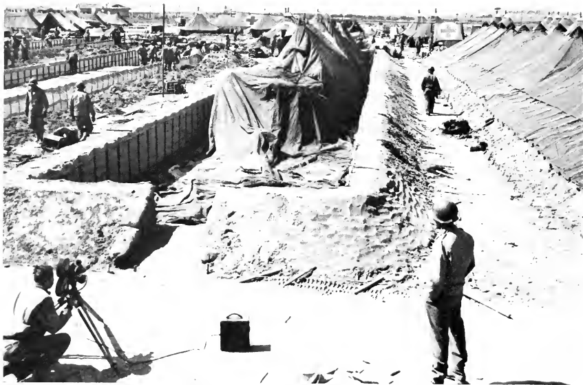
ANZIO HOSPITALS BEING DUG IN AFTER THE GROUND DRIED
