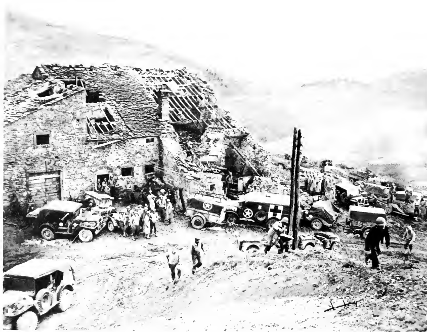
COLLECTING POINT AT PARTIALLY DEMOLISHED HOUSE ON MT. ALTUZZO
