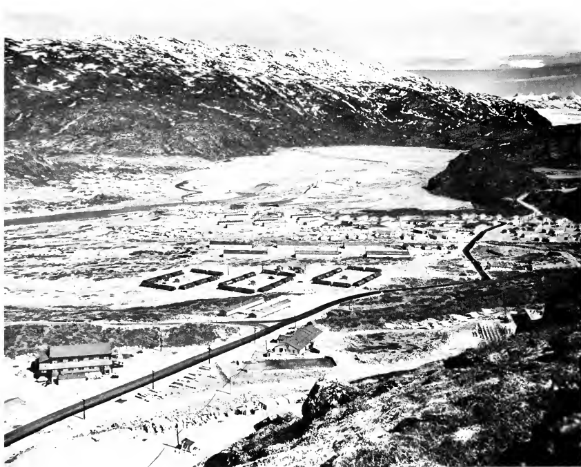
BLUE WEST 1, Narsarsuaq, Greenland, May 1943, with the 188th Station Hospital under construction in right foreground.
