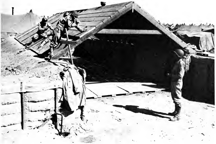
PROTECTING OPERATING TENTS WITH TWO-INCH PLANKS AND SANDBAGS
