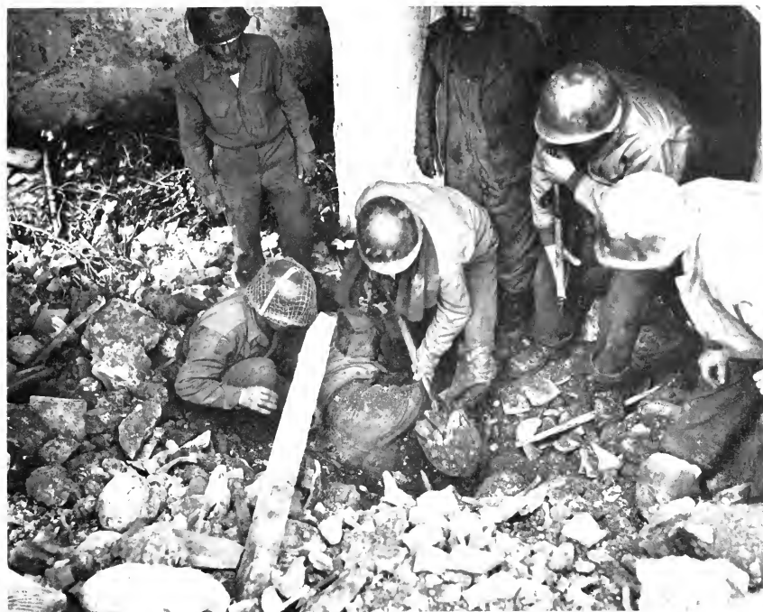
WOUNDED MAN BEING DUG FROM DEBRIS NEAR CASSINO
