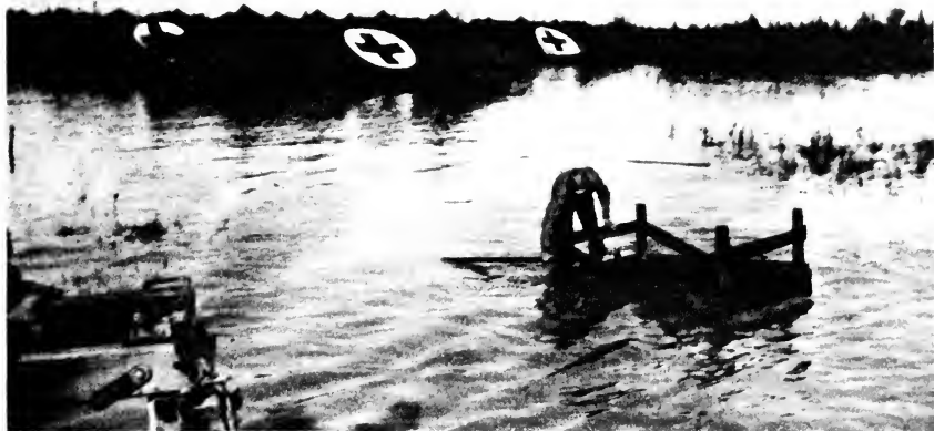
38TH EVACUATION HOSPITAL FLOODED AT PISA, NOVEMBER 1944
