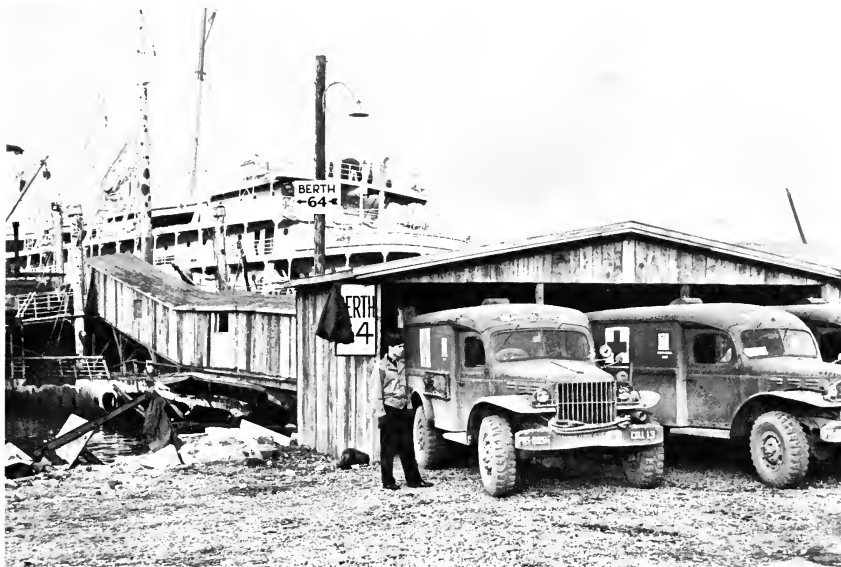
COVERED RAMP TO HOSPITAL SHIP FACILITATED LOADING OF PATIENTS, LEGHORN
