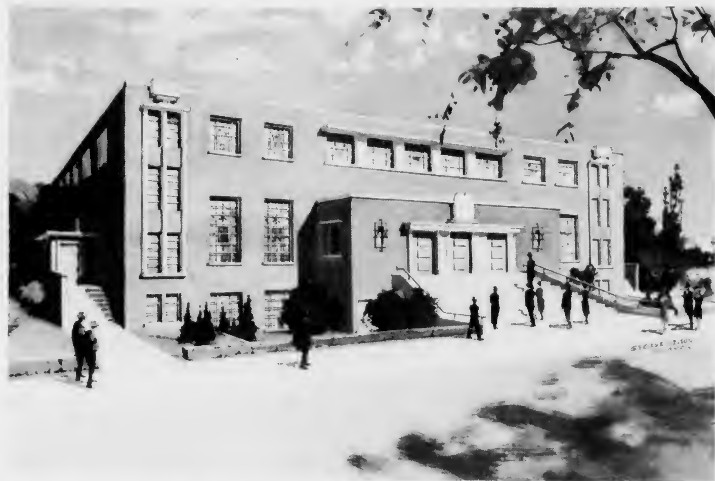
Our new Building - its shell completed - at 91 Bennett Avenue, New York 33.
