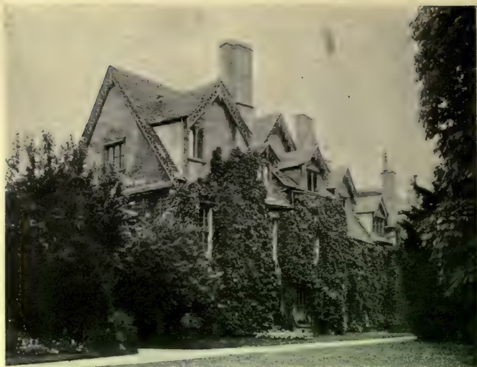
WORCESTER COLLEGE, OXFORD VIEW OF COLLEGE BUILDINGS FROM THE GARDENS
