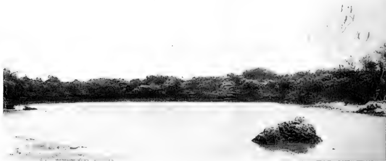
OLD LEDGE DAM AND SPUR, LAGOON SIDE OF WEST COAST OF RANGIROA.
