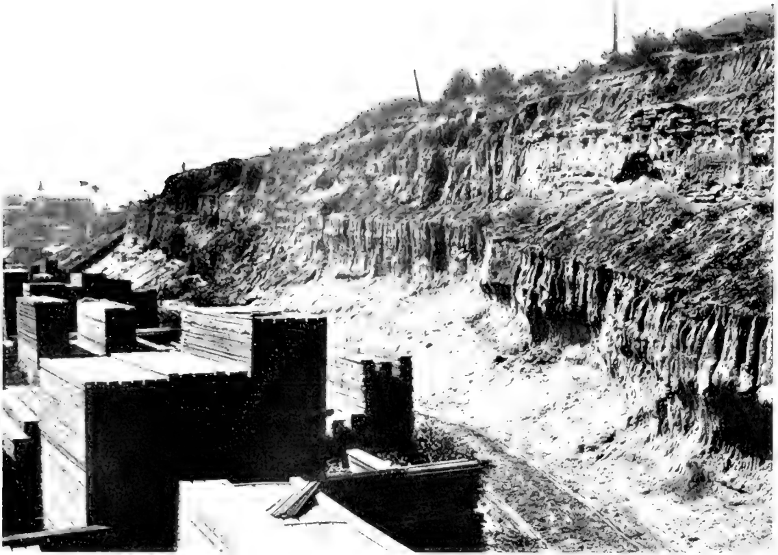
Fig. 1. Erosion of the hillside of the mountain near St. Petersburg, Florida, showing the effect of the erosion on the structure of the hillside. (Photograph by the U. S. Geological Survey, Washington, D. C., in 1911.)
