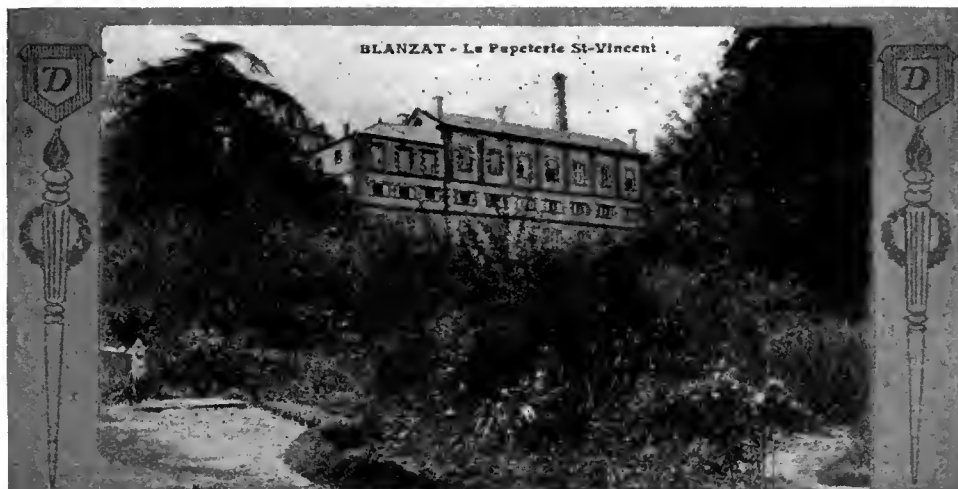
Paper Factory at Blanzat, part of which was occupied by portion of D Bty.
