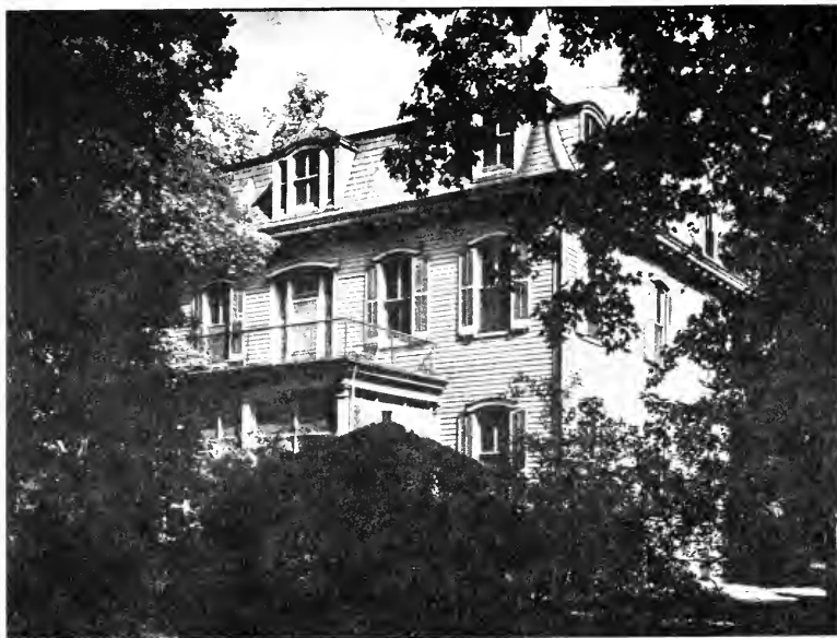
Historic Brickey Home at Prairie du Rocher
