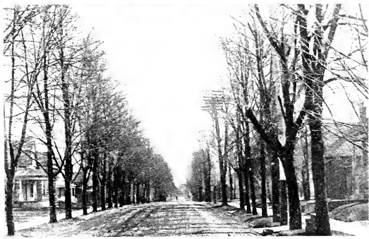
RESIDENCE VIEW, QUINCY, O.
