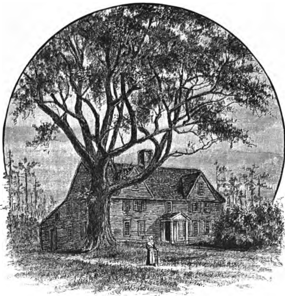
THE OLD ASPINWALL HOUSE. 1
