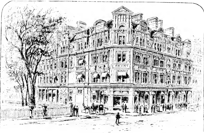
THE GOODWIN BUILDING, CORNER OF ASYLUM AND HAYNES STREETS.
