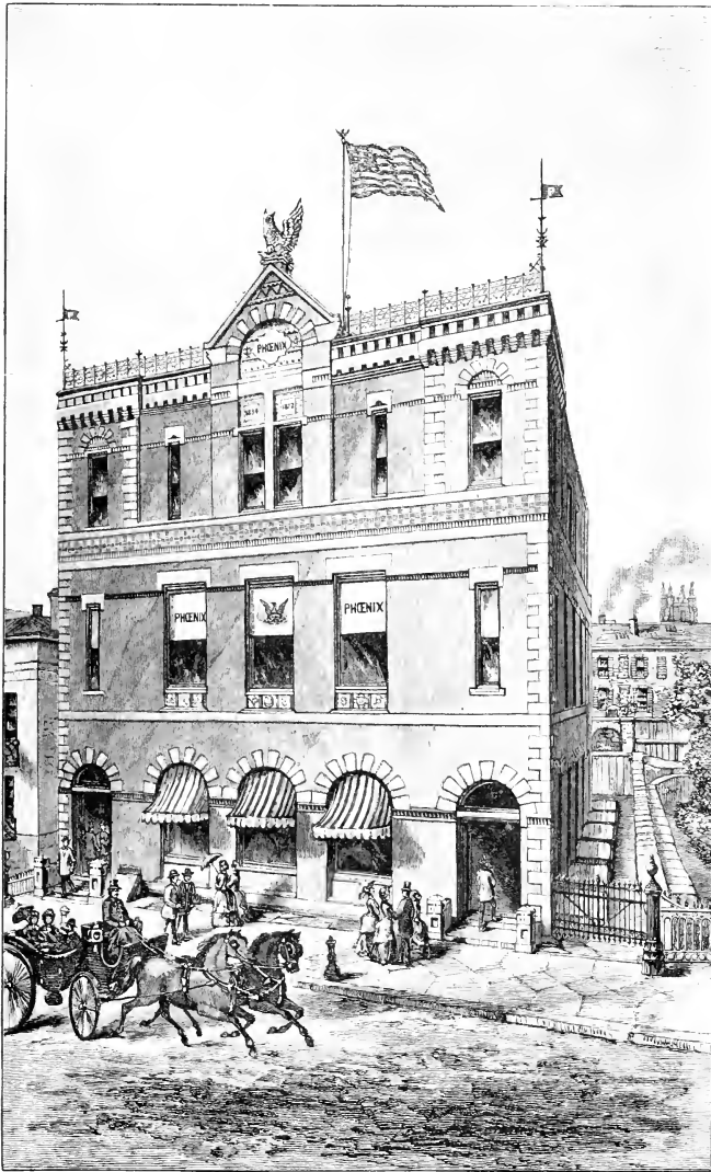
THE PHENIX INSURANCE COMPANY'S BUILDING, ON PEARL STREET.
