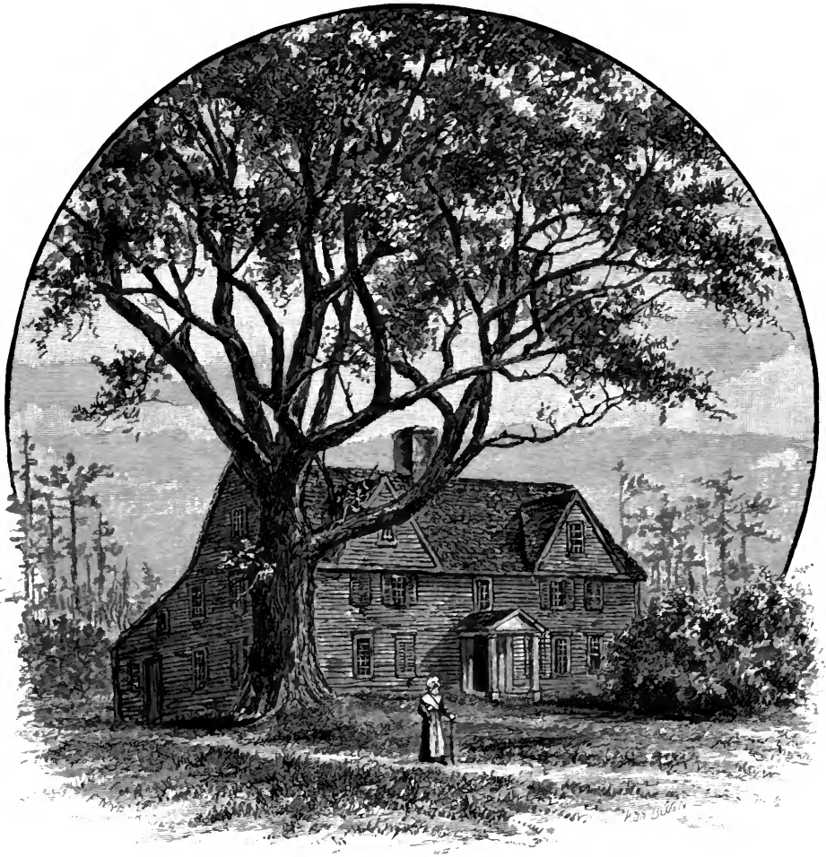
THE OLD ASPINWALL HOUSE. 1
