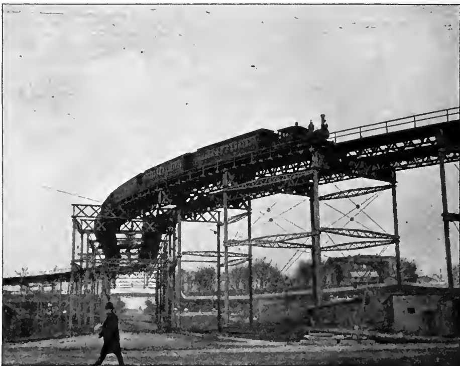
THE ELEVATED RAILWAY.
