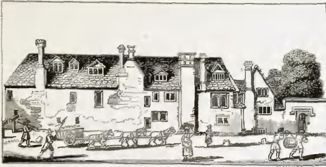
OLD BUILDINGS ; REDUCED FROM LOGGAN.
