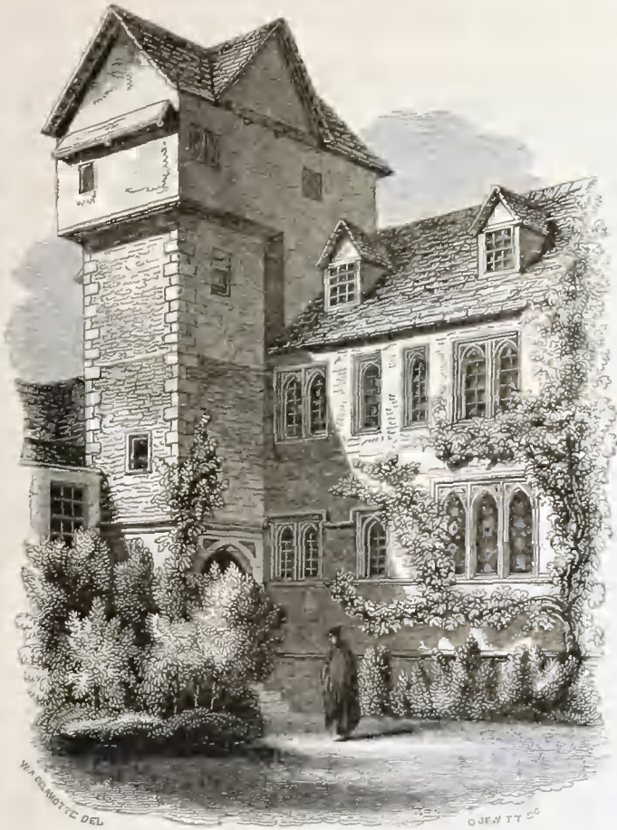
BELL TOWER, &c.
