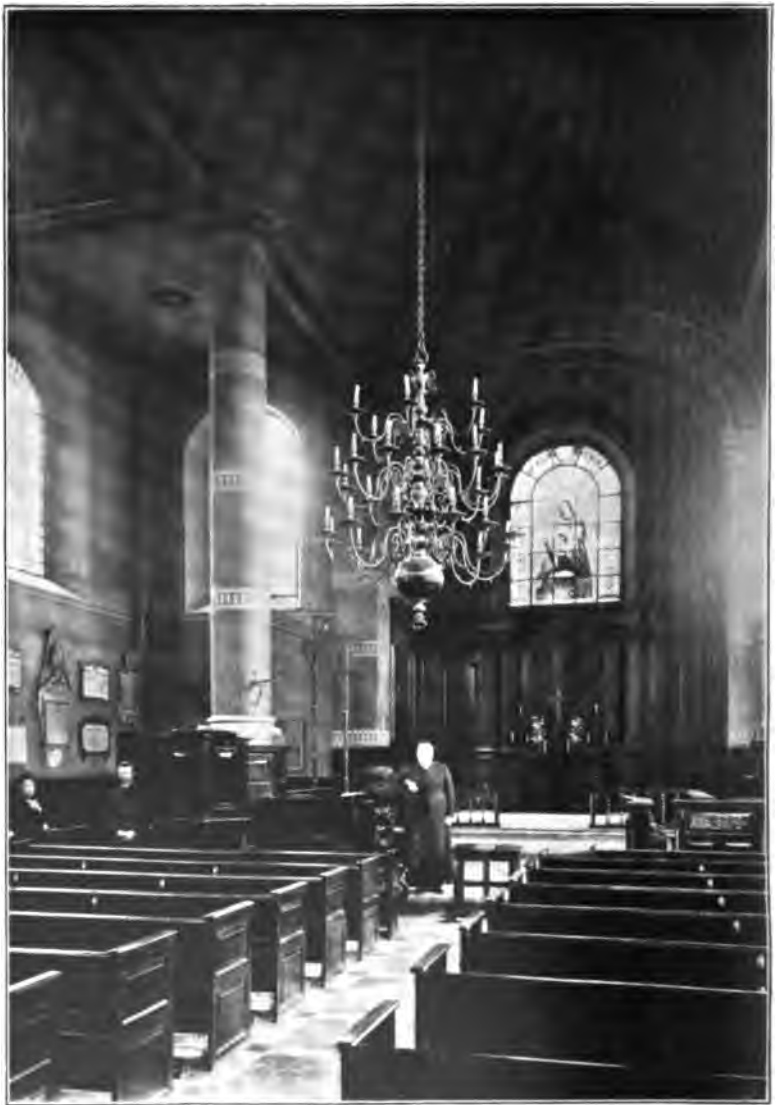
Interior of St Mary, Rotherhithe. (Nave.)
