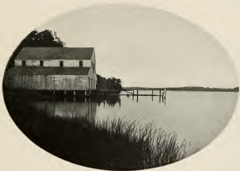
UNIVERSITY BOATHOUSE, ERECTED 1871-72
