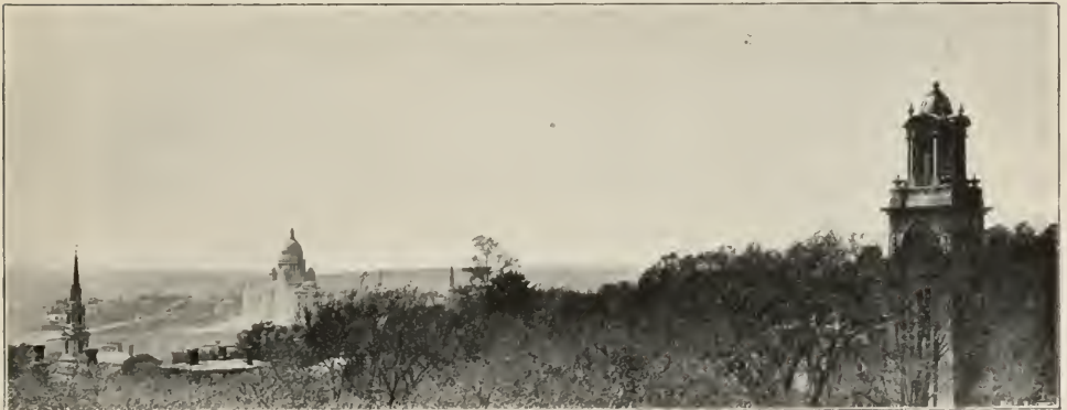
VIEW FROM THE ROOF OF UNIVERSITY HALL
