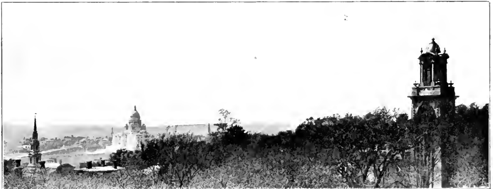
VIEW FROM THE ROOF OF UNIVERSITY HALL
