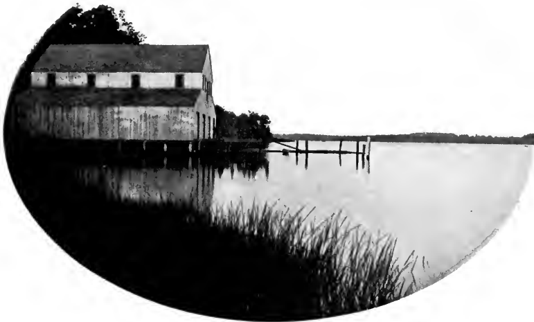
UNIVERSITY BOATHOUSE, ERECTED 1871-72
