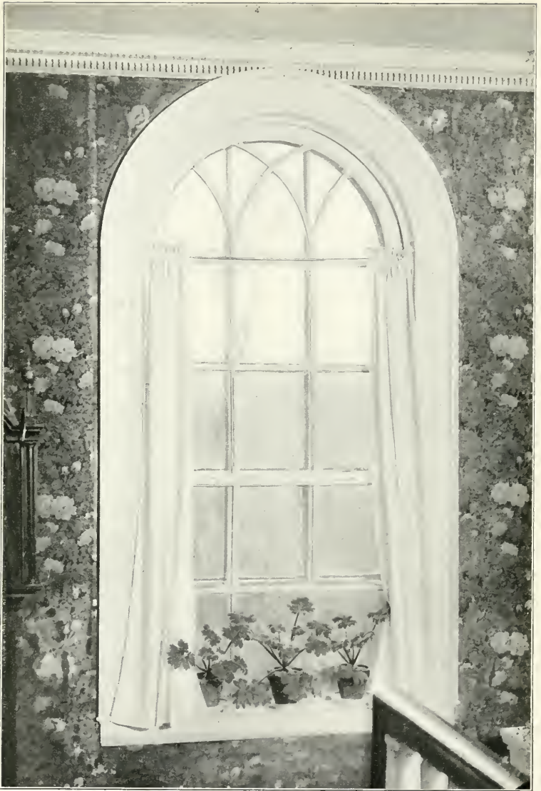
The Palladian window in the Cook-Oliver house has been inserted at the landing on the front stairs
