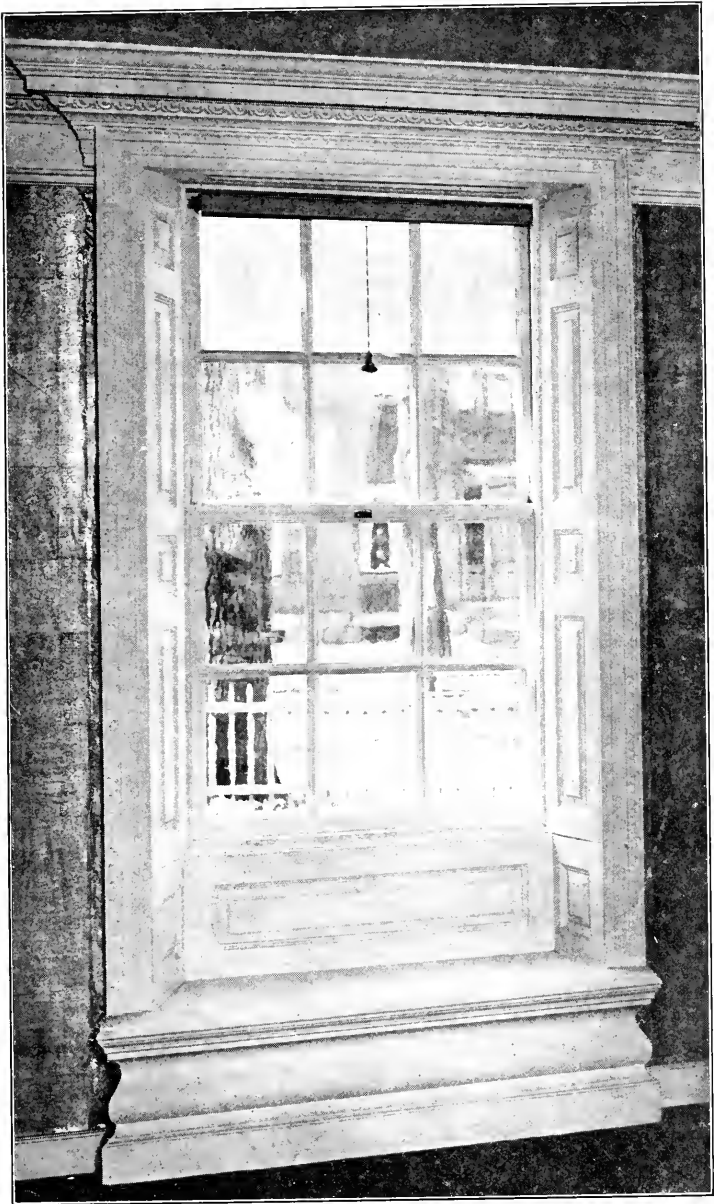
The embrasured window with its twelve panes is of the Georgian type, showing folding shutters and window seat
