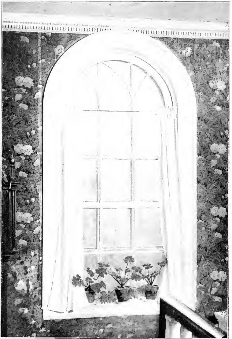
The Palladian window in the Cook-Oliver house has been inserted at the landing on the front stairs
