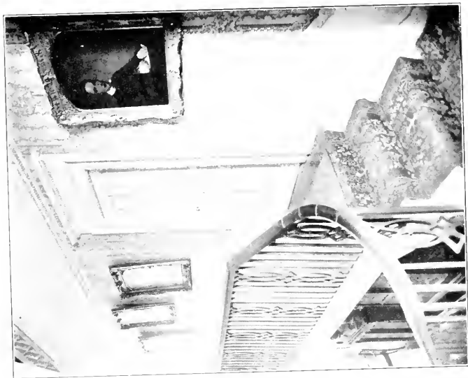
An interesting detail in the Pierce-Nichols house — a Chippendale balustrade
