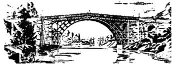
PLATE 46. The first structural experiment with cast iron was the bridge over the Severn at Coalbrookdale, opened in 1779 : the last great cast iron structure was built seventy two years later, and was Paxton's Crystal Palace.
