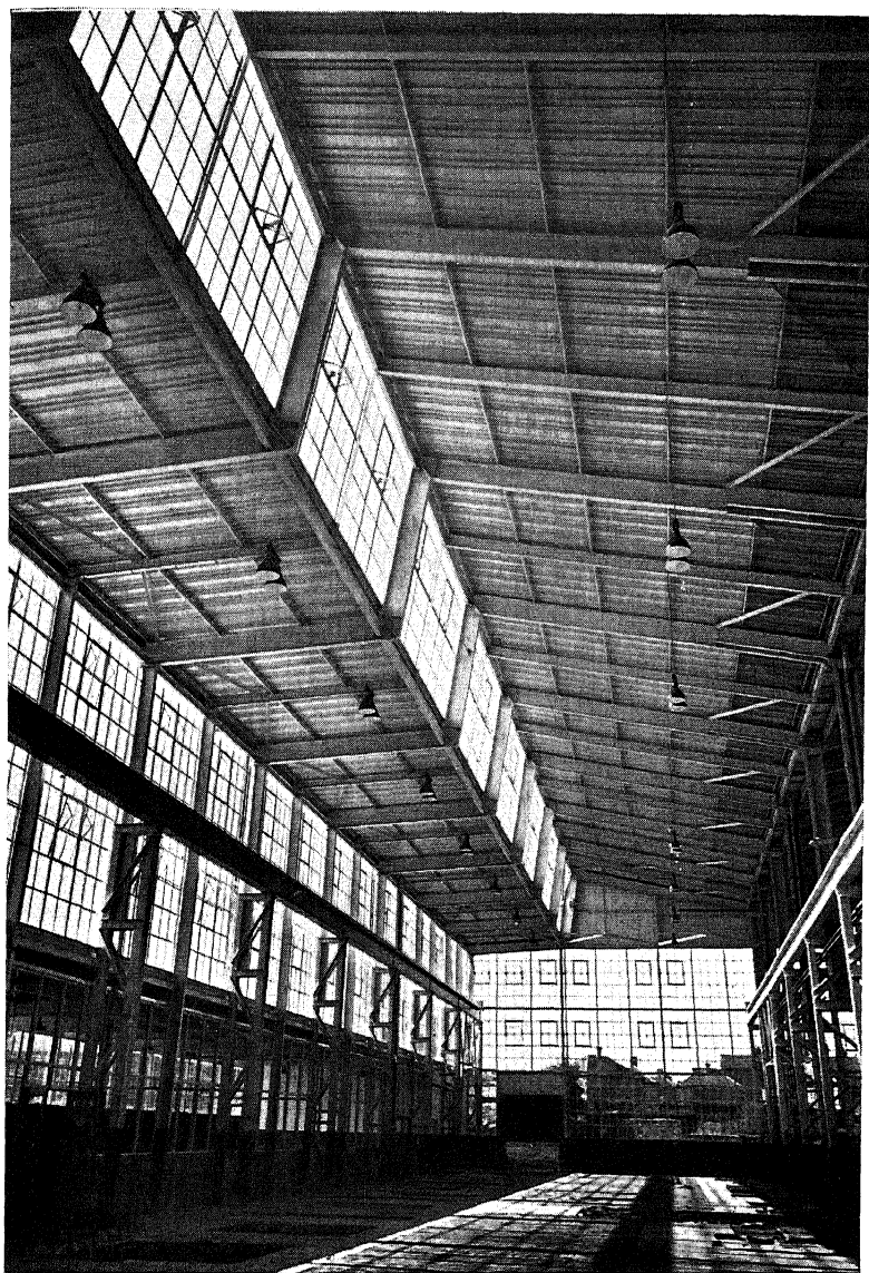
PLATE 51. The metal and glass structural technique of modern industrial building which has been derived from the original example of the Crystal Palace. This is an interior in a factory at Wolverhampton, designed by Howard Crane for Bayliss, Jones & Bayliss Limited.
