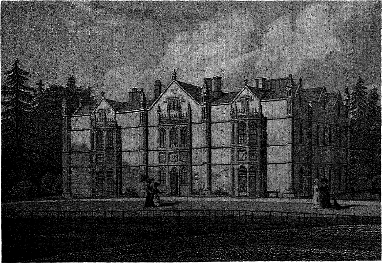
Adlestrop Park, Gloucestershire, as it appeared in the early nineteenth century. The bay windows ascending through two storeys have a Gothic flavour ; but the house, to which various additions had been made, is not unduly fussed and fretted with applied ornamental features. It preserves a true Georgian serenity.
