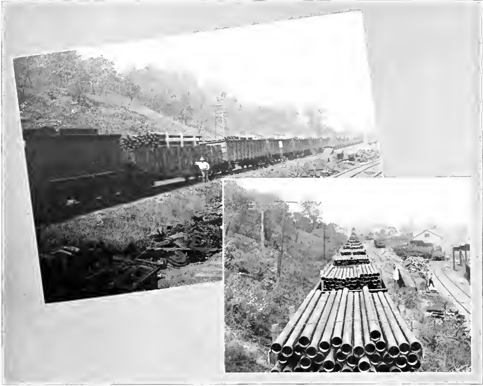
TRAIN LOAD OF PIPE BEING SHIPPED TO ATLAS SUPPLY CO., Muskogee
