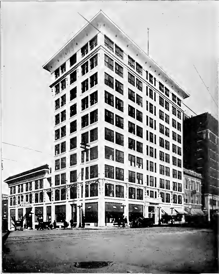
R. T. DANIEL OFFICE BUILDING, Tulsa. Built by Van Horn & Son
