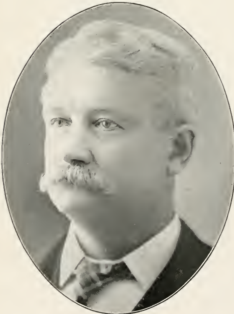
R. MONTGOMERY, GENERAL MANAGER THE YOUNGSTOWN GAS & ELECTRIC CO.
