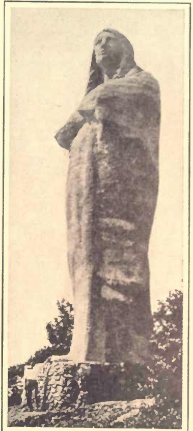
BLACK HAWK, BY LORADO TAFT A concrete work of gigantic proportions, overlooking Rock River, Illinois.
