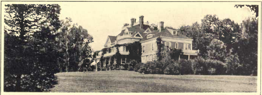
ALEXANDER GRAHAM BELL'S SUBURBAN RESIDENCE AT WASHINGTON, D. C.
