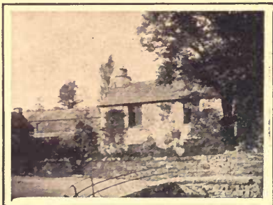
DOVE COTTAGE At Town End, Grasmere.
