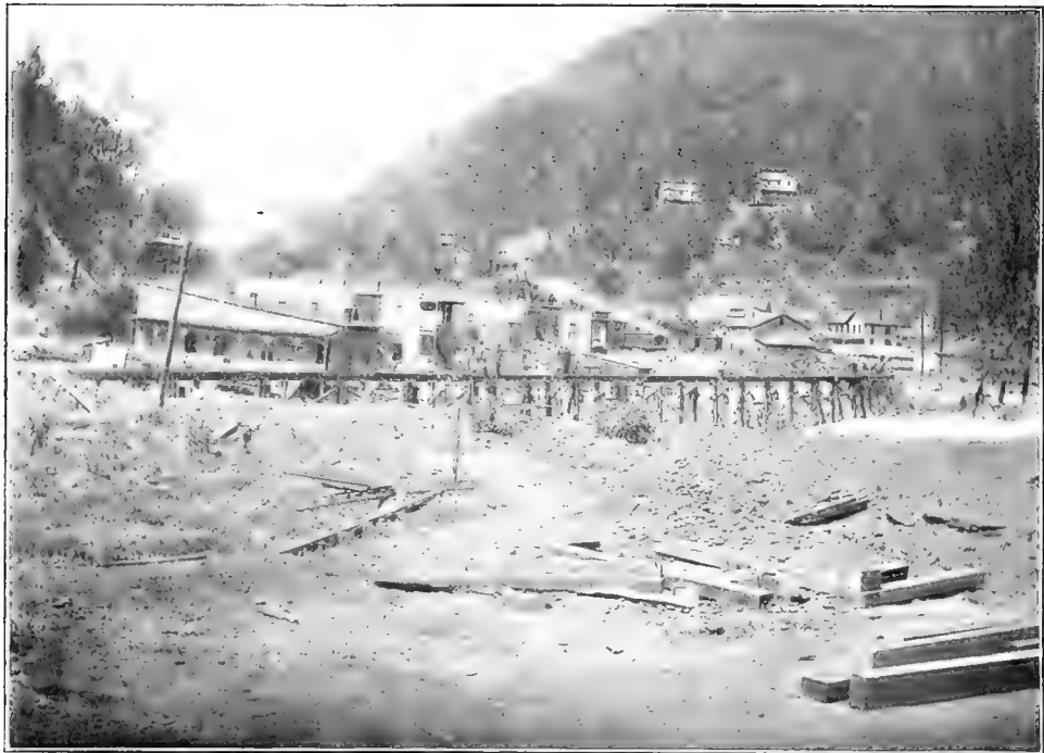
(B) FLOOD DAMAGES TO RAILROAD AND MINING SETTLEMENT, KEYSTONE, W. VA., 1901.
