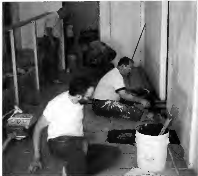
Bremen Brethren lay tile in Caimito's community center.
