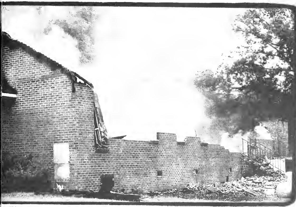
Alabama burning. An early morning fire destroyed the Rising Star Baptist church in Greensboro, Ala. The fire is still under investigation.
