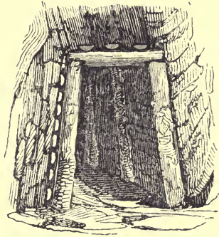
Timbering in a level with solid rock on one side.
