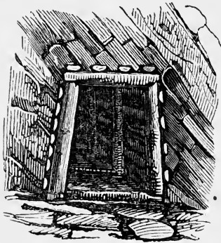
Timbering in a level in a yielding rock.
