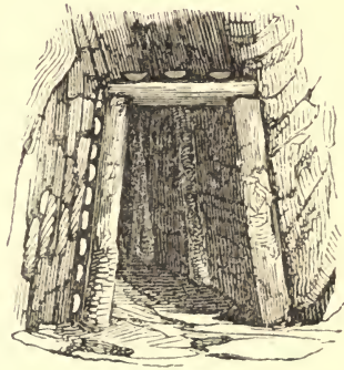
Timbering in a level with solid rock on one side.
