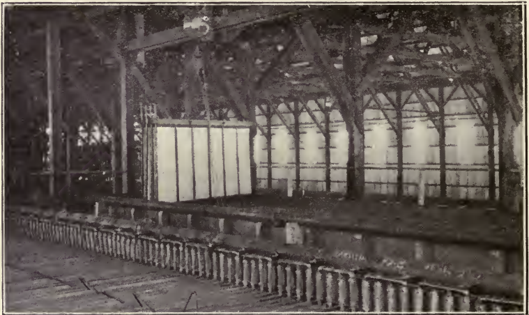
Fig. 88. BUTTERS FILTER TANKS.
