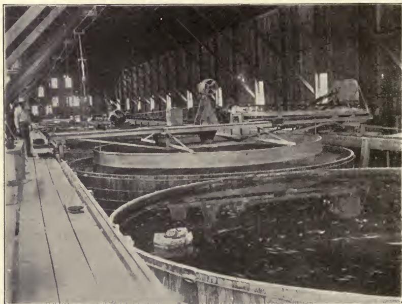
Fig. 87b. SAND DISTRIBUTOR, BLAISDELL SYSTEM.
