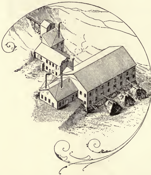
Fig. 81. VIEW OF FIFTY-TON CYANIDE PLANT.
