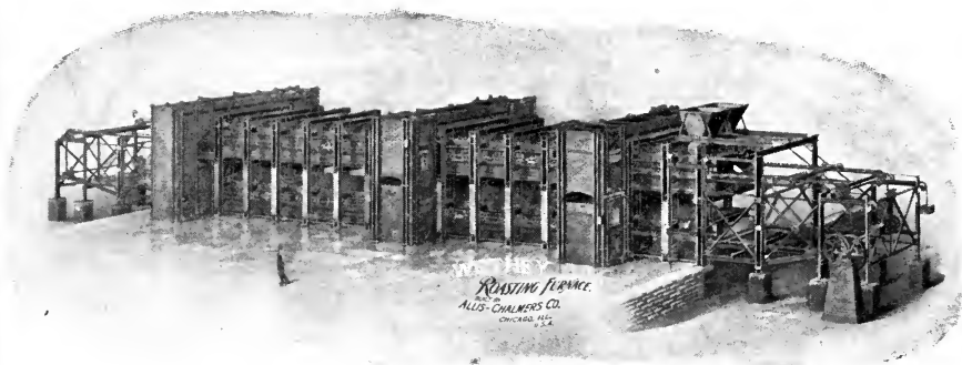
Fig. 36. VIEW OF WETHEY ROASTING FURNACE.
